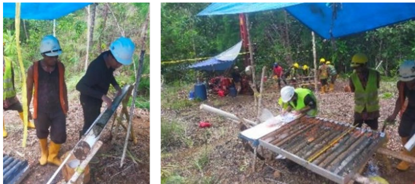
Geotech drilling activities
