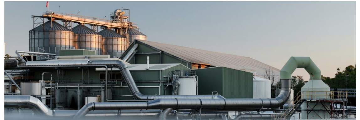
GrainCorp oilseed crush plant, Numurkah, Victoria
