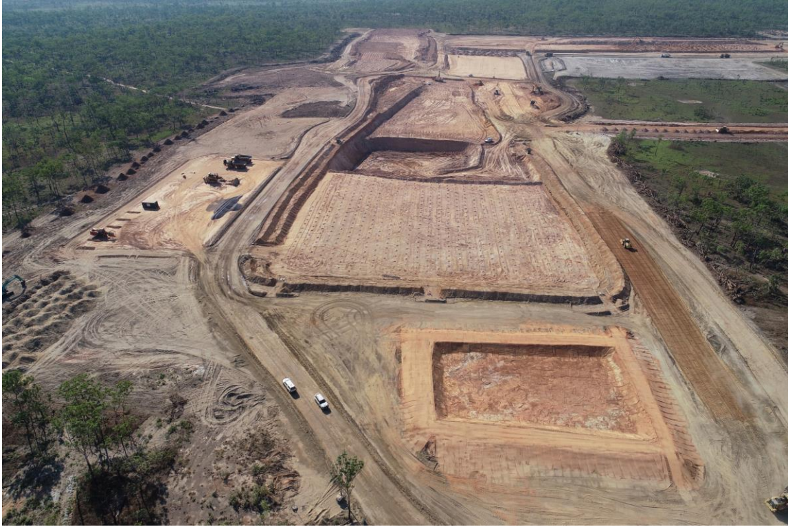
BP33 aerial view early September – box cut excavation commences.
