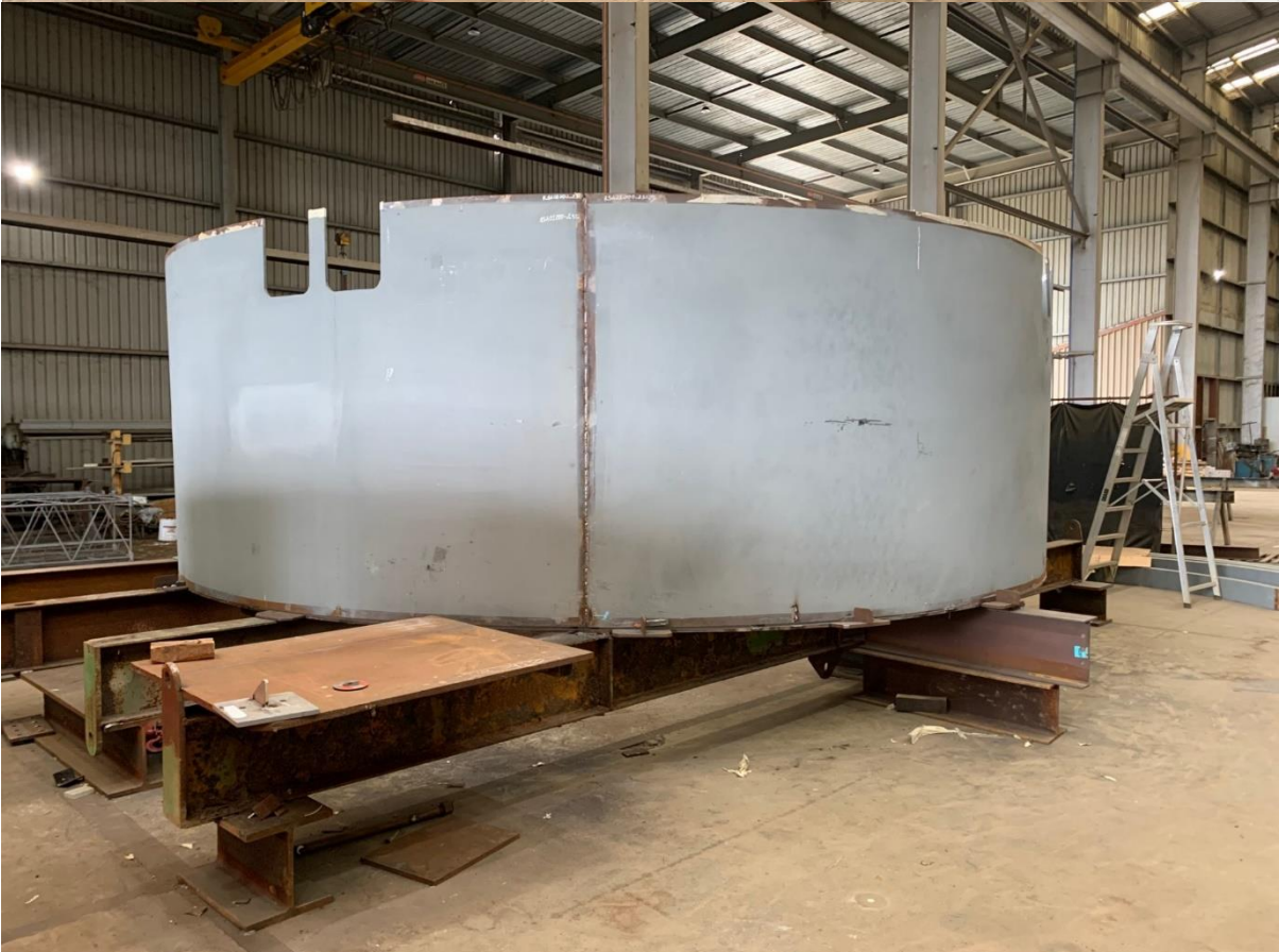
Figure: Workshop Fabrication of Spray Roaster Reactor Shell
