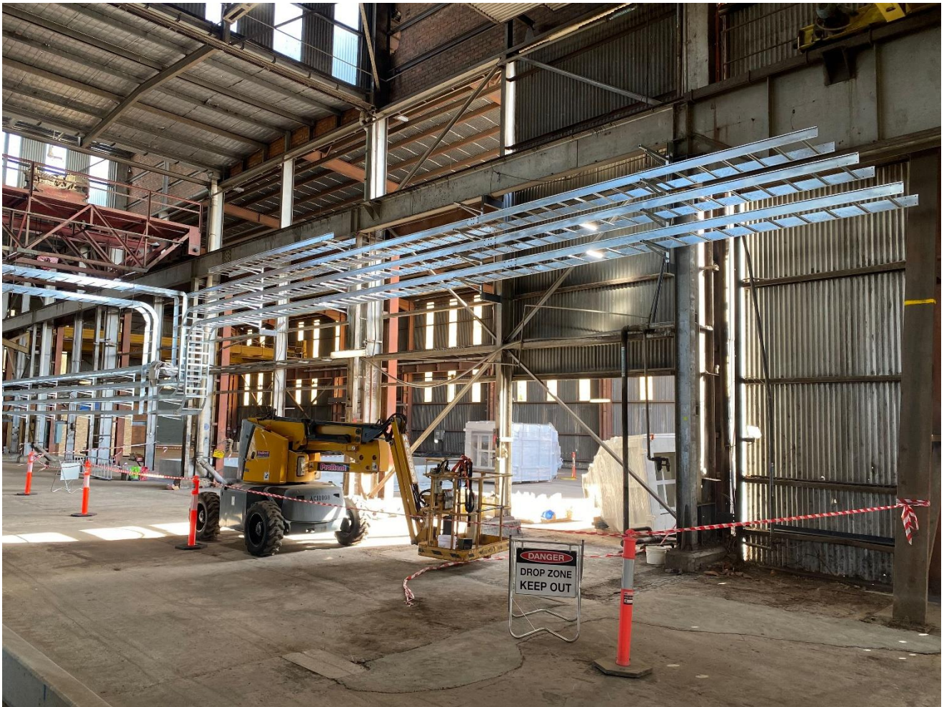
Figure: Erection of Pipe Rack and Supports
