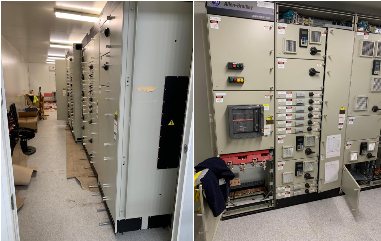
Figure: Installation of MCC into Switch rooms
