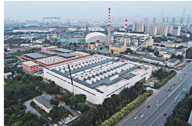
Worlds largest Vanadium battery Dalian Province China, 100MW (400MWh) and enough power to meet demand from 200,000 residents
