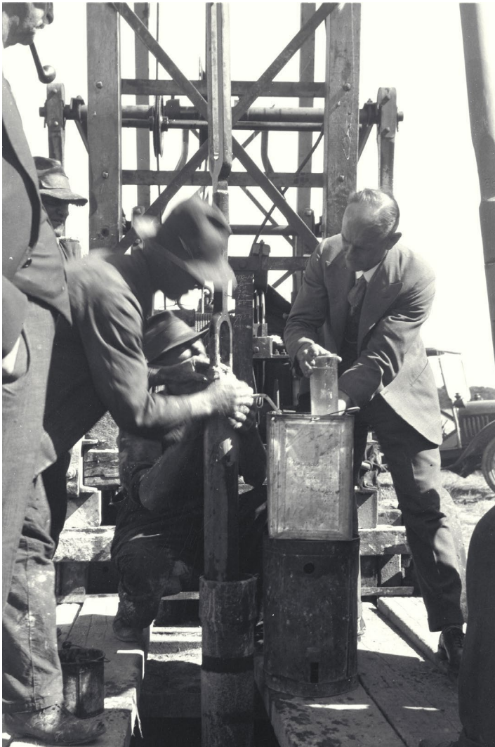
Gas sampling whilst drilling – Ramsay Oil Bore
