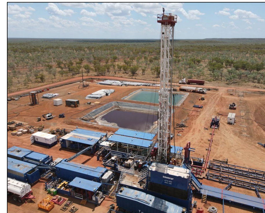
SLB 185 Rig drilling Carpentaria-3H in EP187
