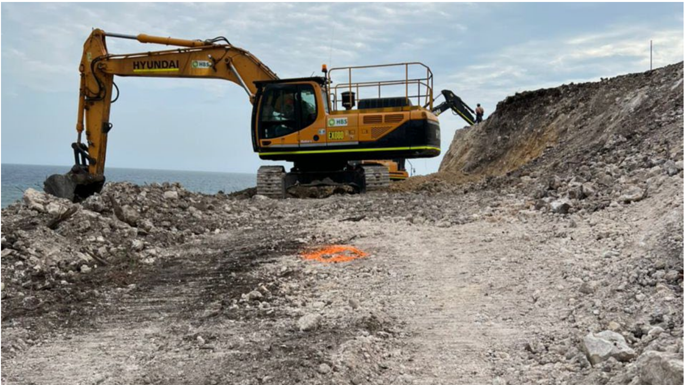
Landside of Wharf under Construction
