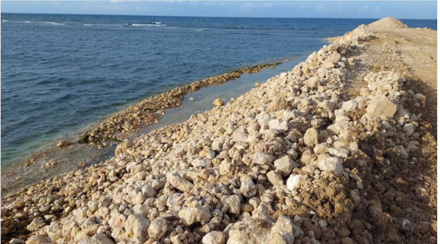
Inner Core of Wharf under Construction
