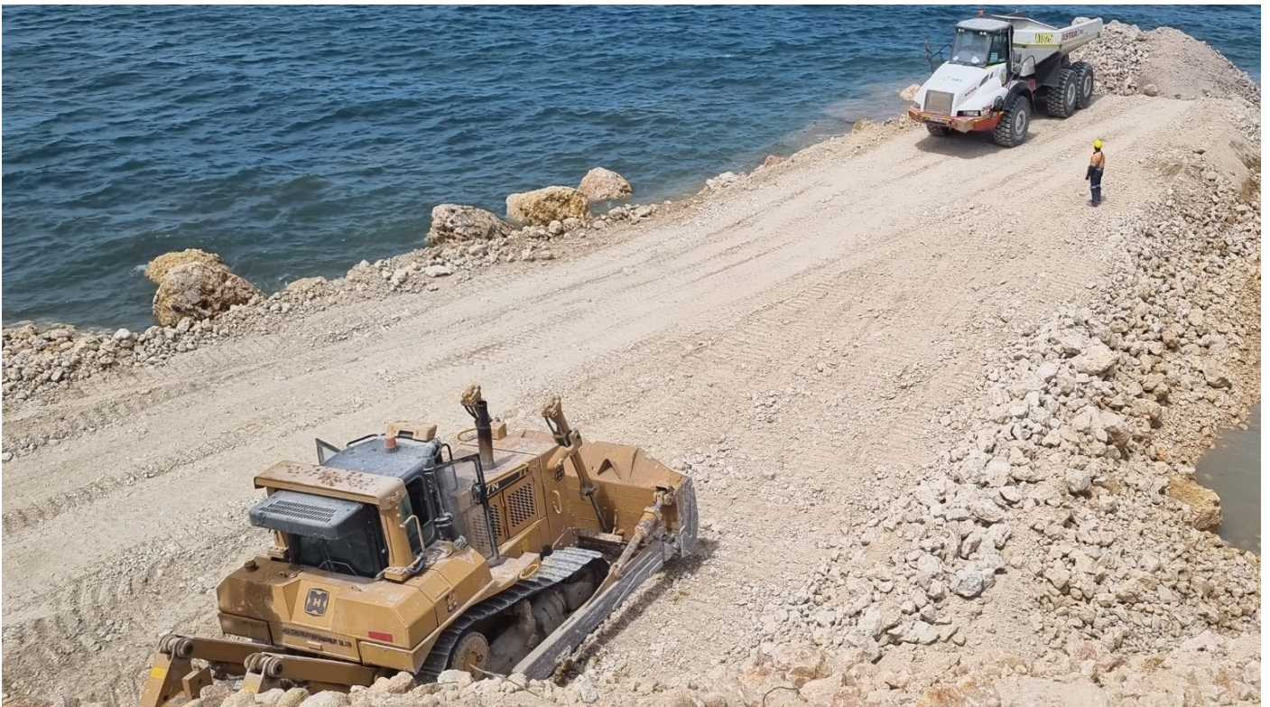
Wharf under Construction
