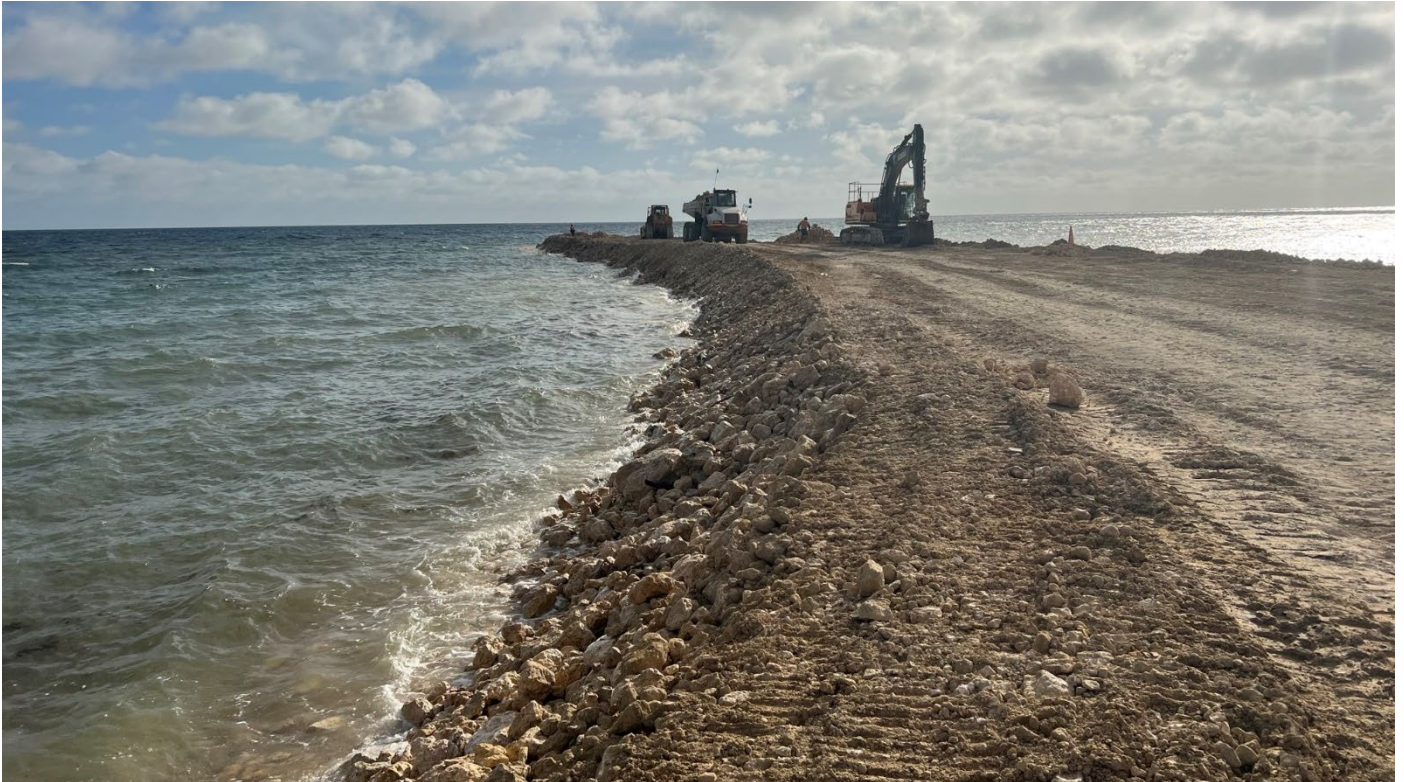
Inner Core of Wharf Almost at Full Chainage
