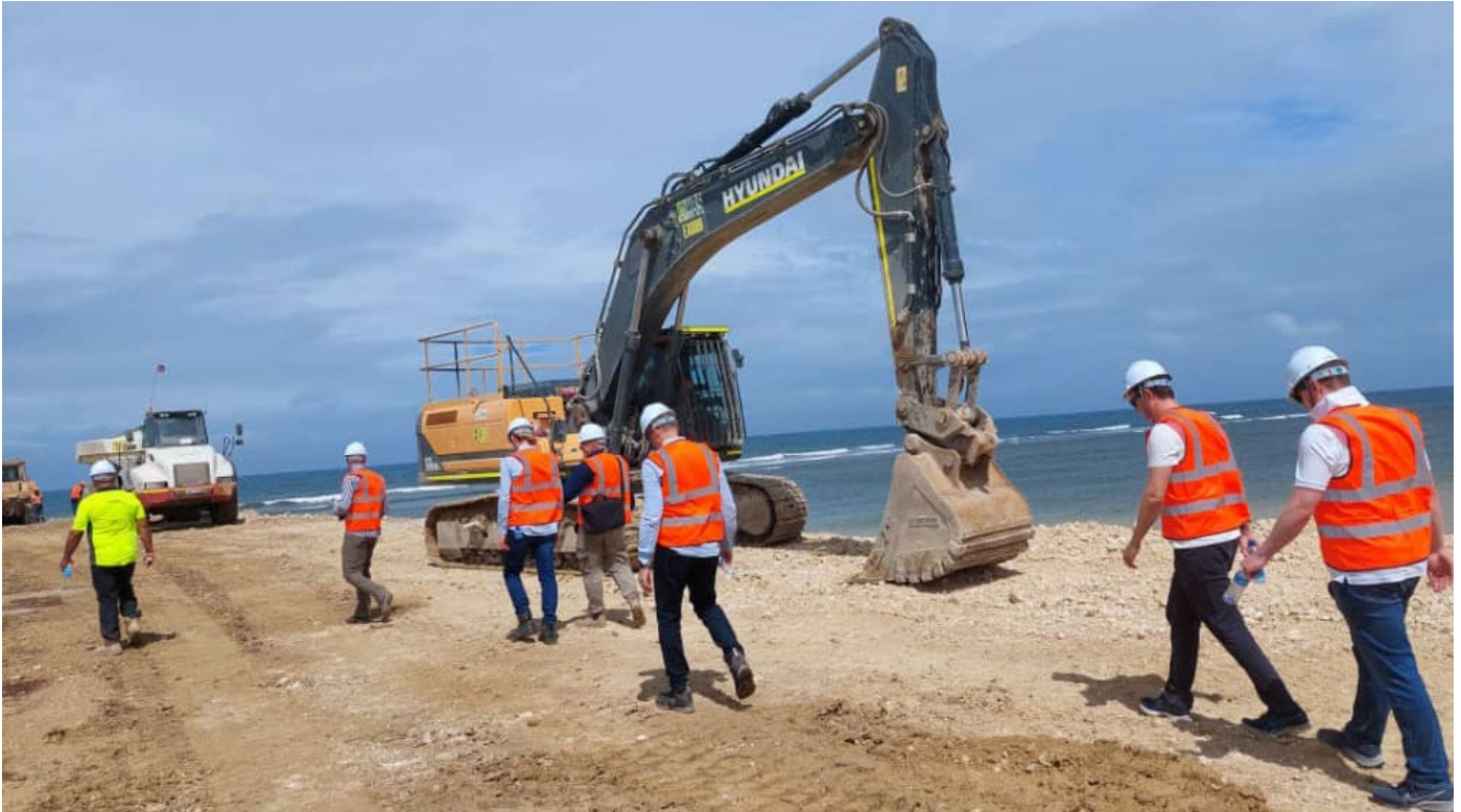
Vision Blue inspecting Wharf Construction Progress
