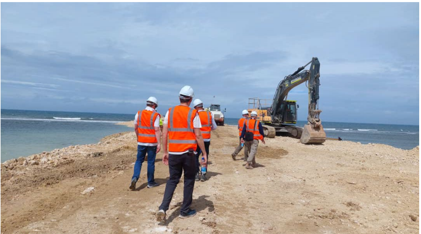
Vision Blue inspecting Wharf Construction Progress
