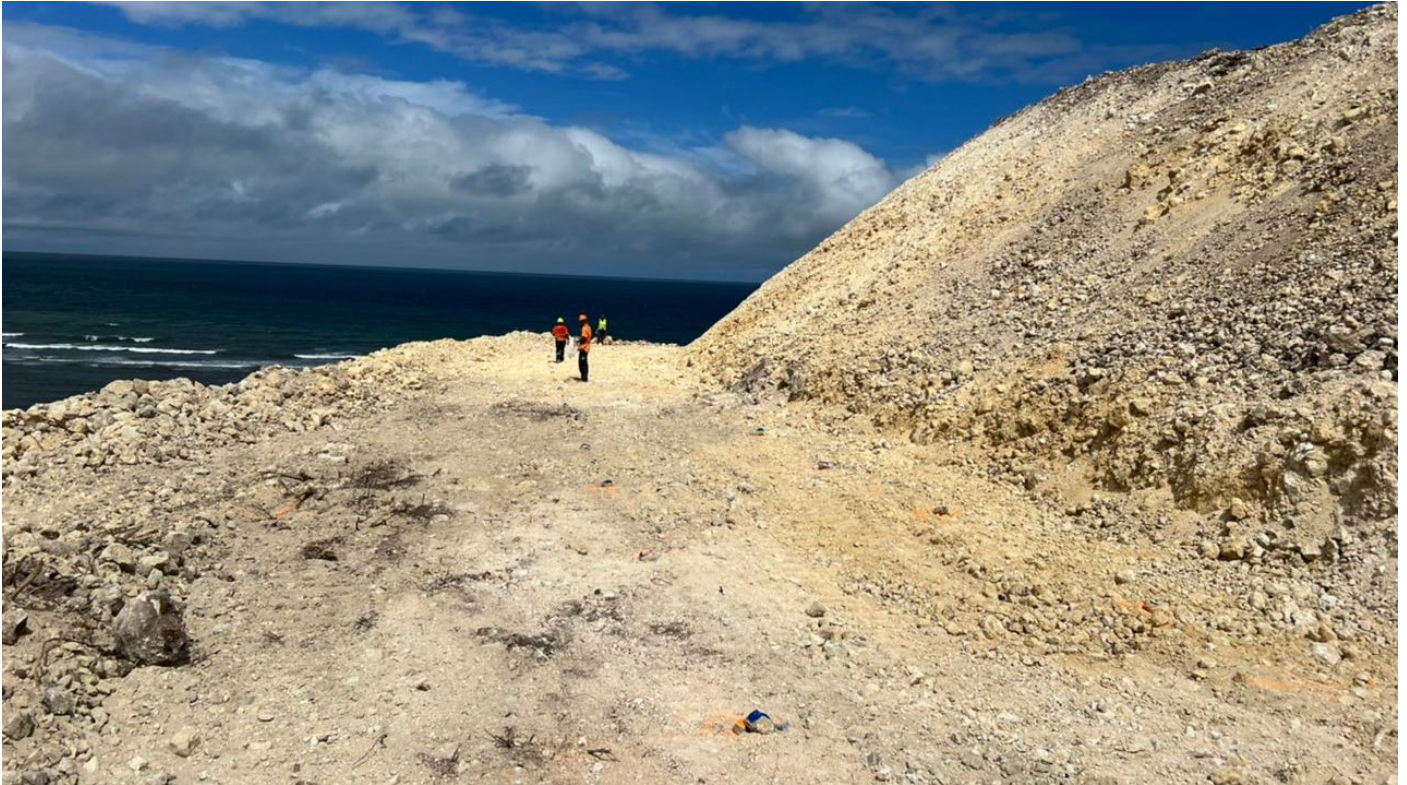
Wharf under Construction
