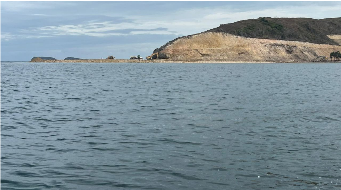
Side profile of Wharf Construction Site
