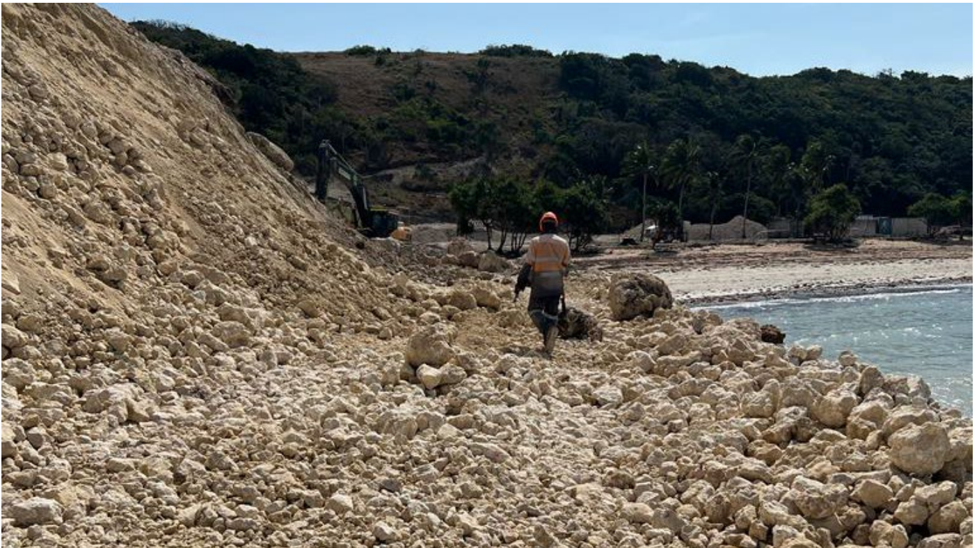
initial Wharf Construction Activities
