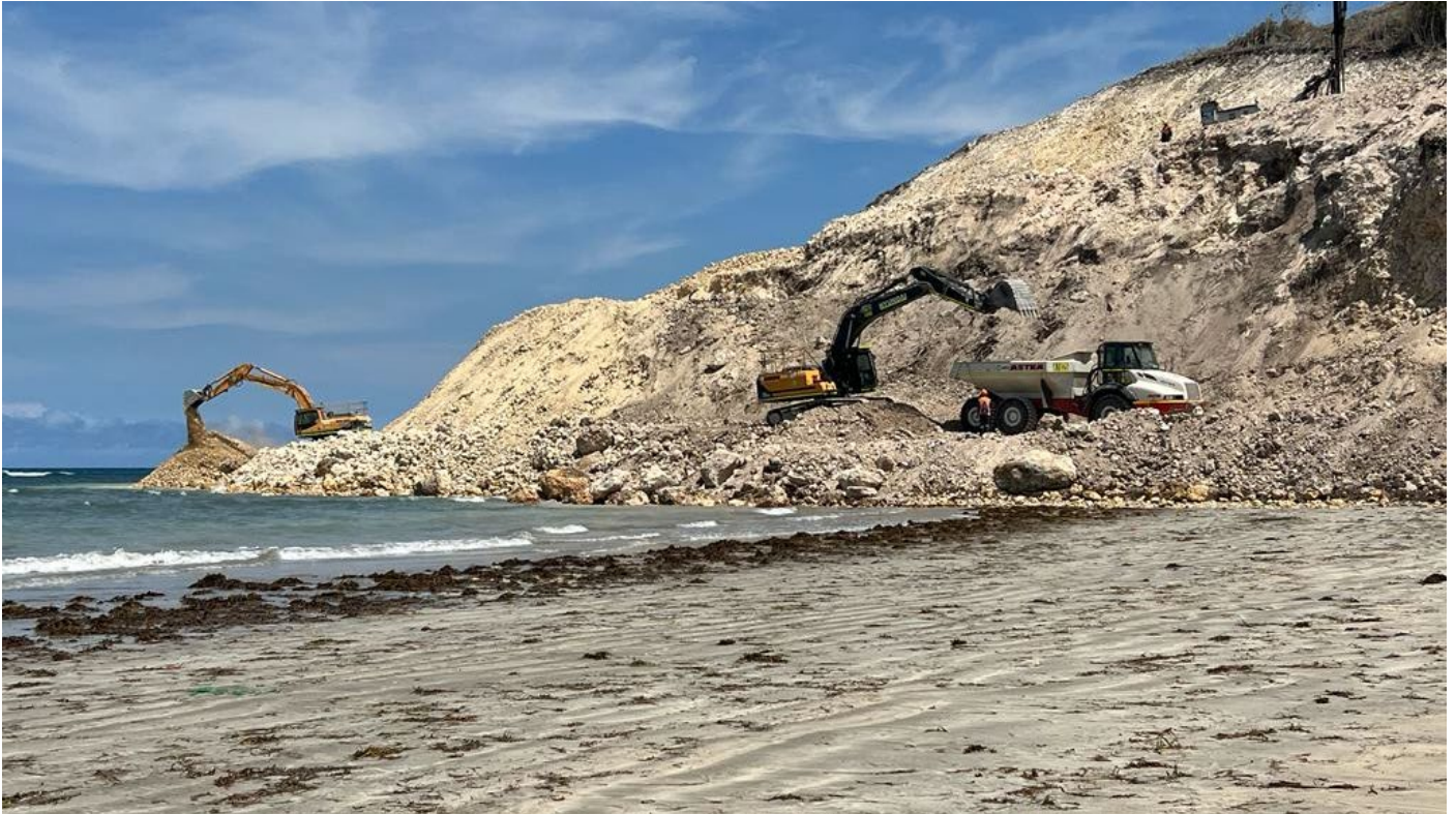
Landside of Wharf under Construction
