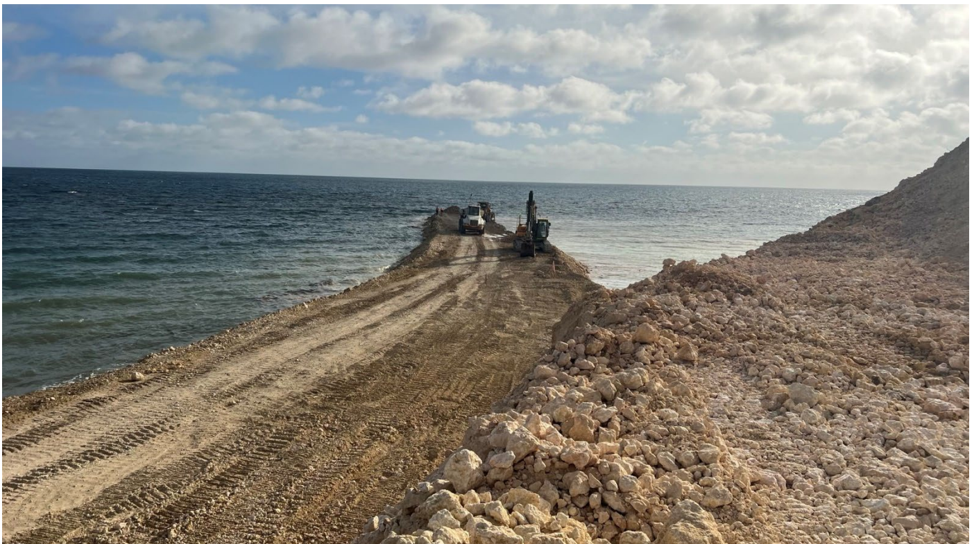
Wharf under Construction
