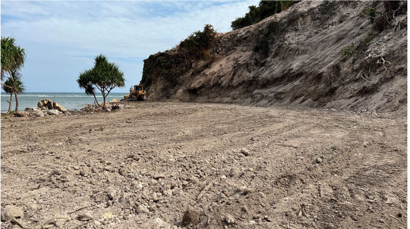
Landside Preparation for Wharf Construction
