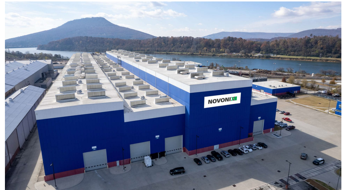
Riverside Facility in Tennessee
