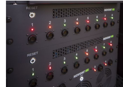
Diagnostic tools and performance testing
