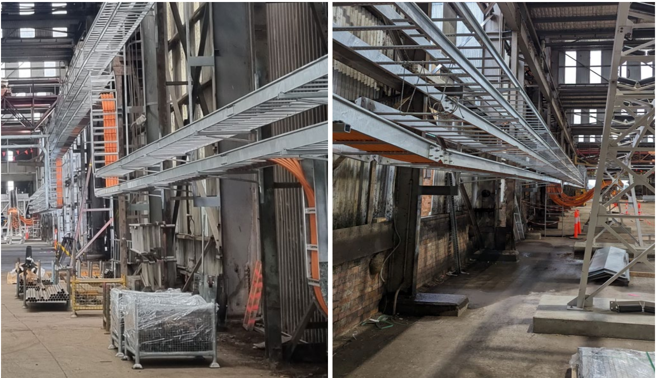
Figure: Cable Installation in Cable Trays
