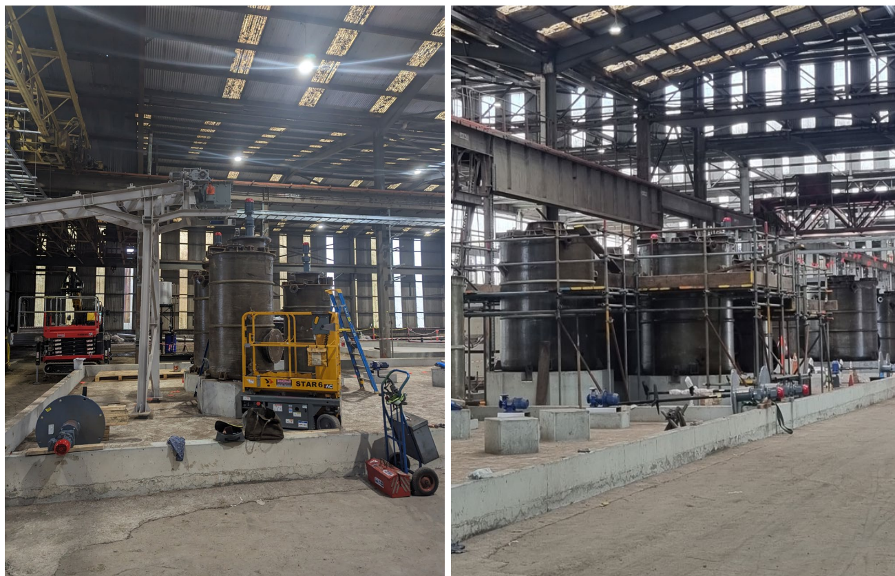
Figure: Erection of Agitators in Hydromet Tanks (left) and Scaffolding for Pipe Installation (right)
