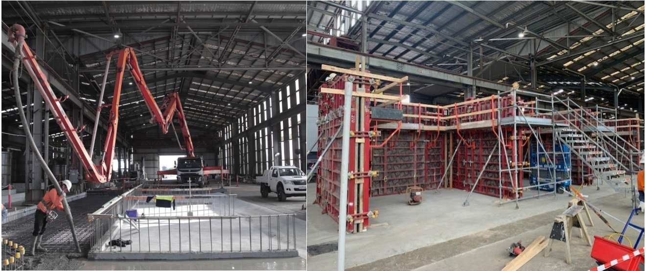
Figure: Filtration Area Base Concrete Pour (left) and Filtration Area Wall Pour (right)
