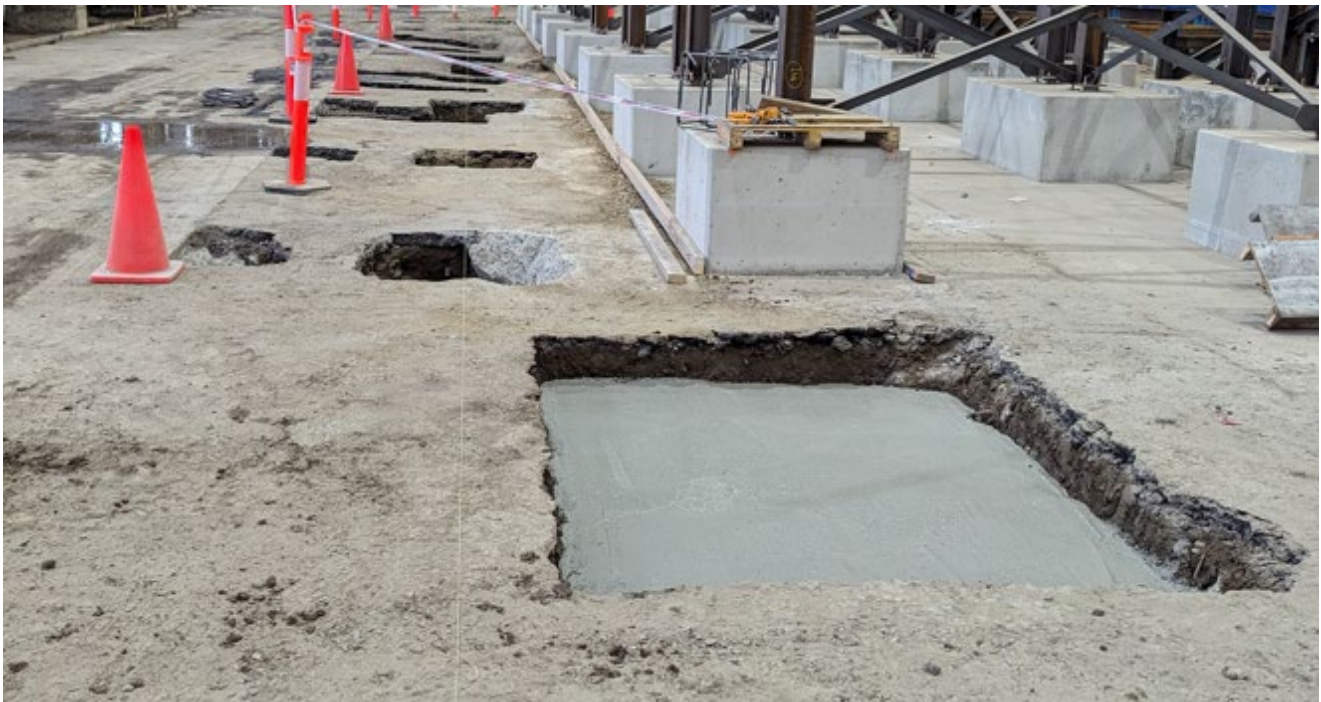
Figure: Foundations for Furnace Automation
