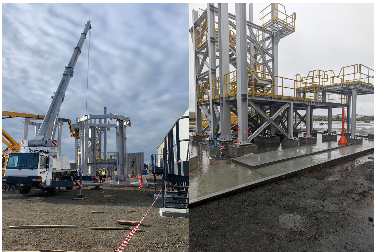
Figure: Erection of Spray Roaster Structural Steelwork
