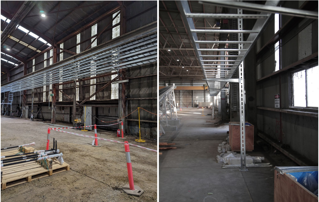
Figure: Main pipe racks (left) and Furnace Area pipe racks (right)
