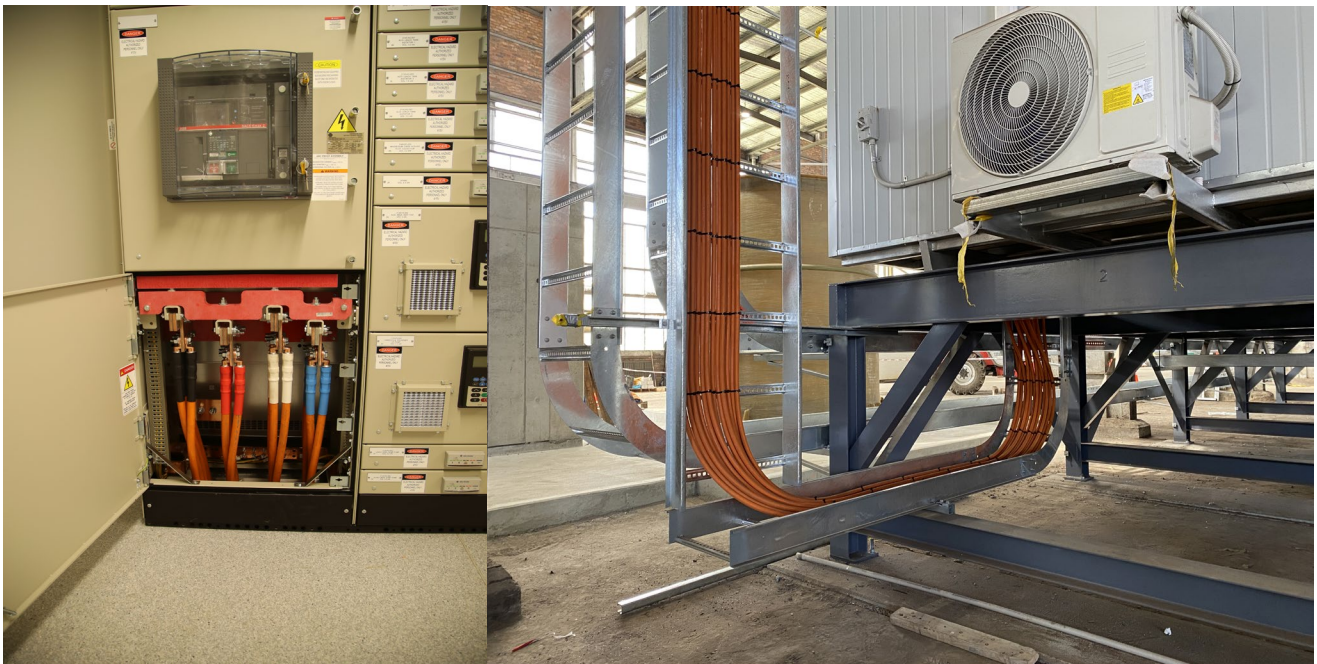
Figure: Termination of main incomers (left) and cabling between switchrooms (right)
