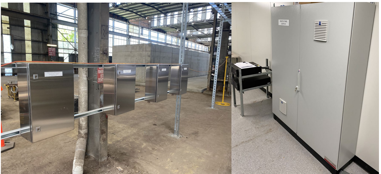
Figure: Installation of instrument junction boxes (left) and control cabinets (right)
