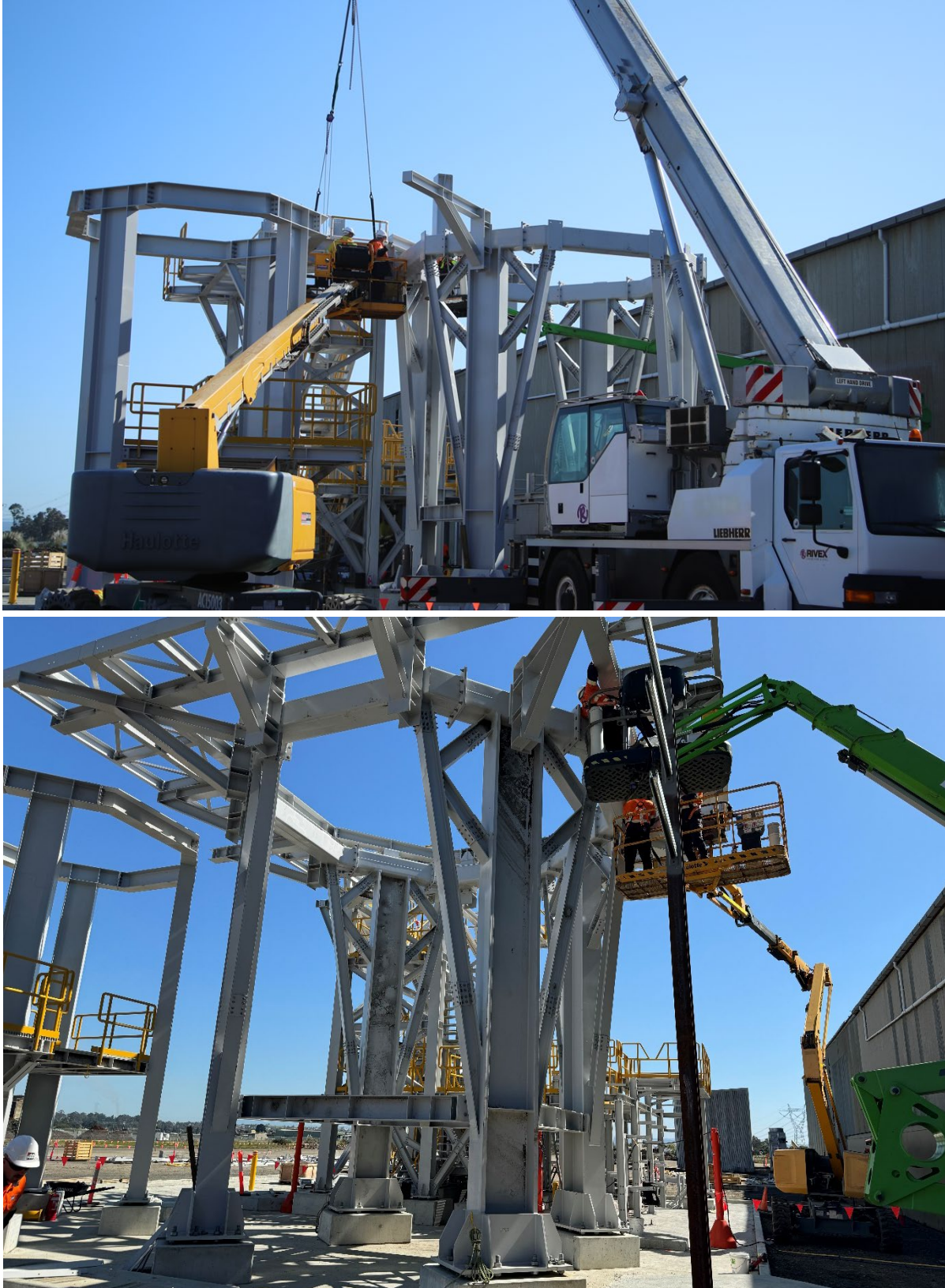
Figure: Spray Roaster structural steelwork erection
