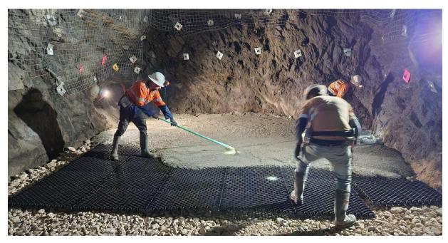
Figure 1 Preparing an underground drilling platform
