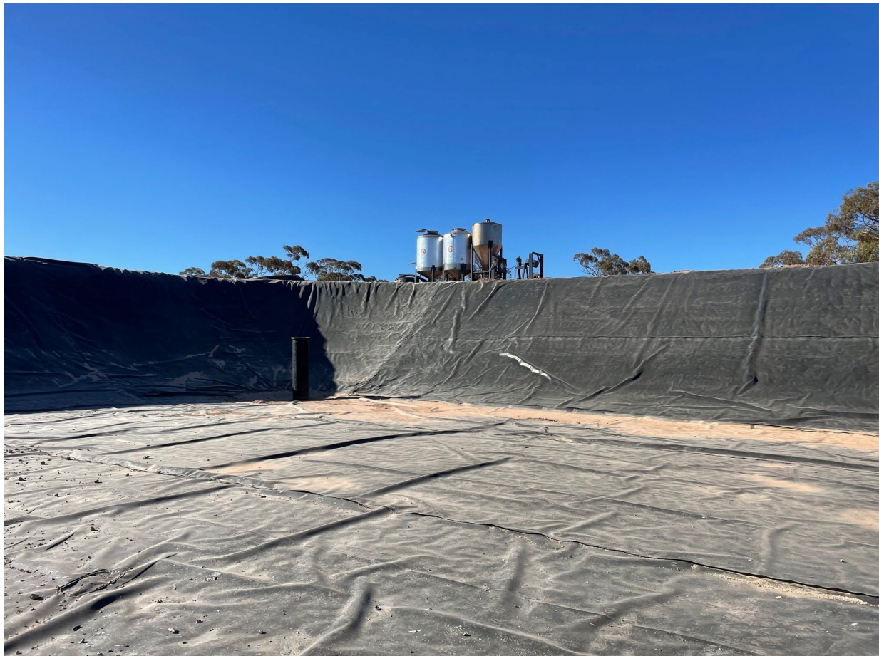
Figure 1: An Eastern Goldfields example of a vat leach pad under construction (source: Lamington Minerals)
