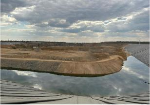
Figure 2: Wises Dam liner installation
