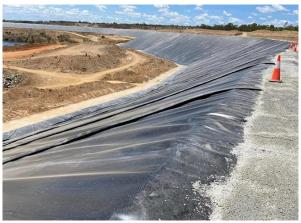
Figure 3: Wise Dam liner installation
