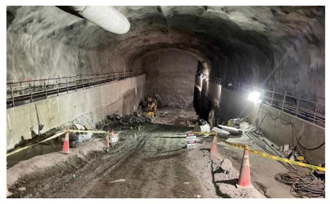
Figure 1: Powerhouse Cavern excavation
