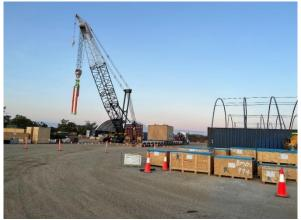
Figure 5: Unloading of one of the main inlet valves at the laydown area on site
