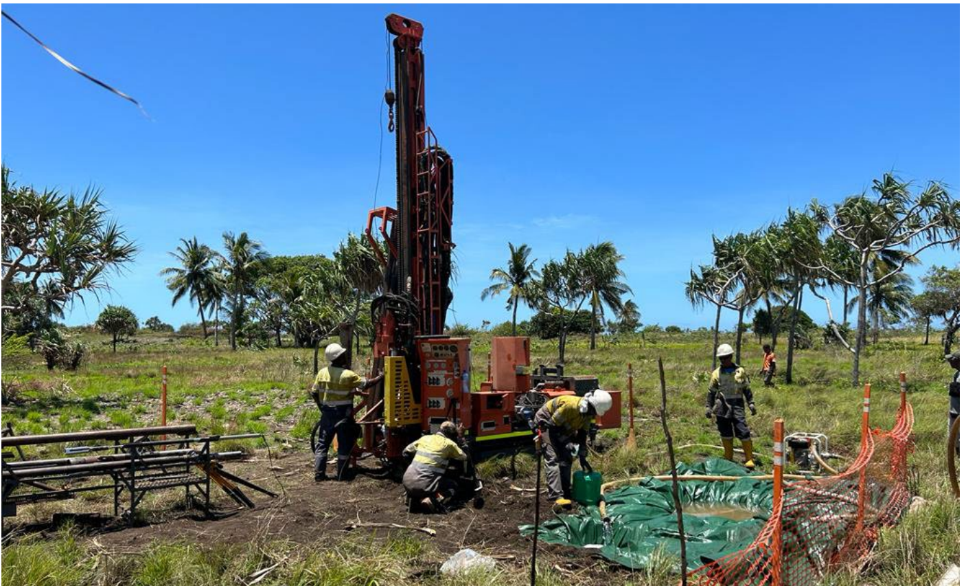
Geotechnical Drill Rig being Setup
