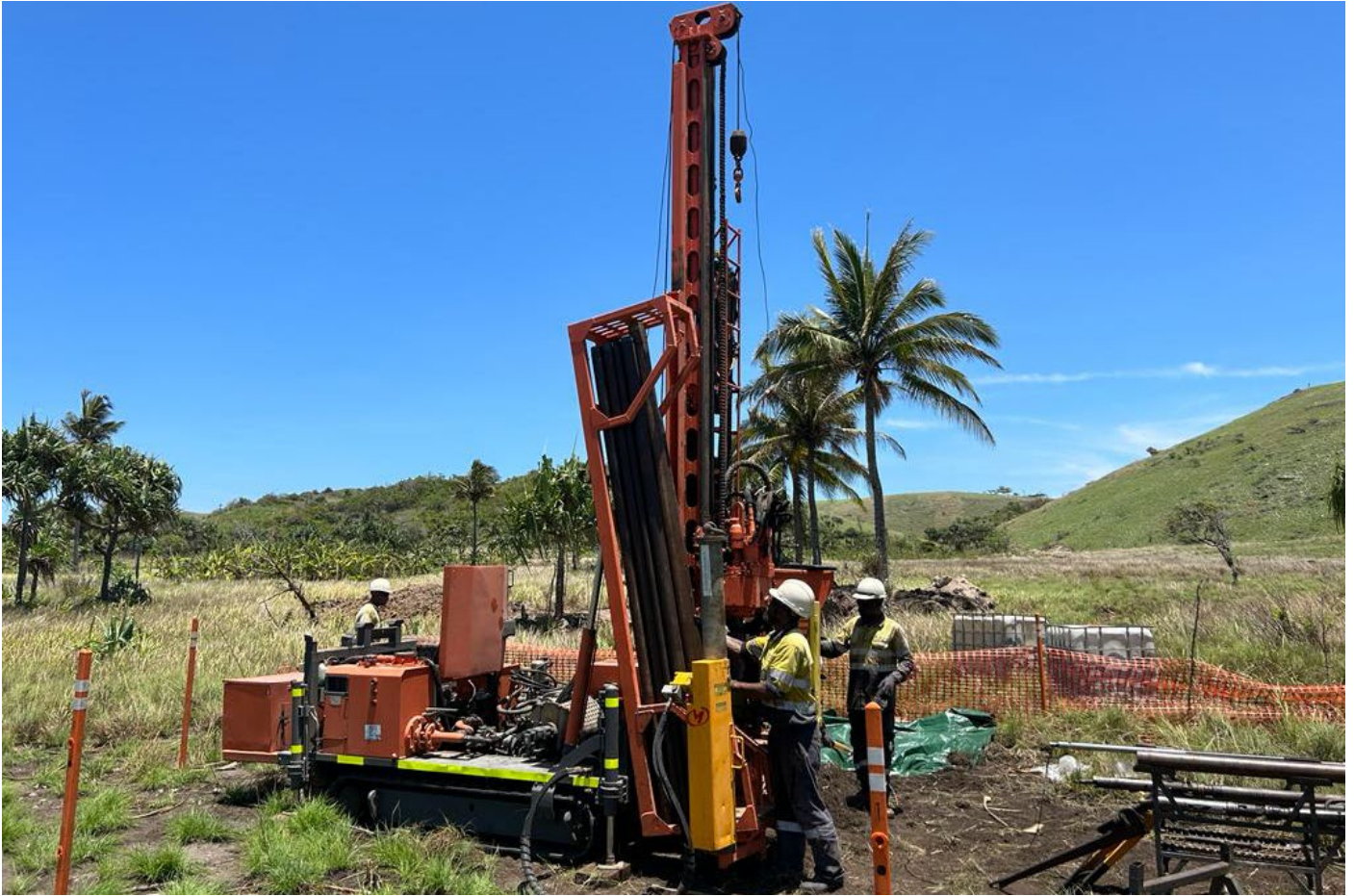
Geotechnical Drill Rig being Setup
