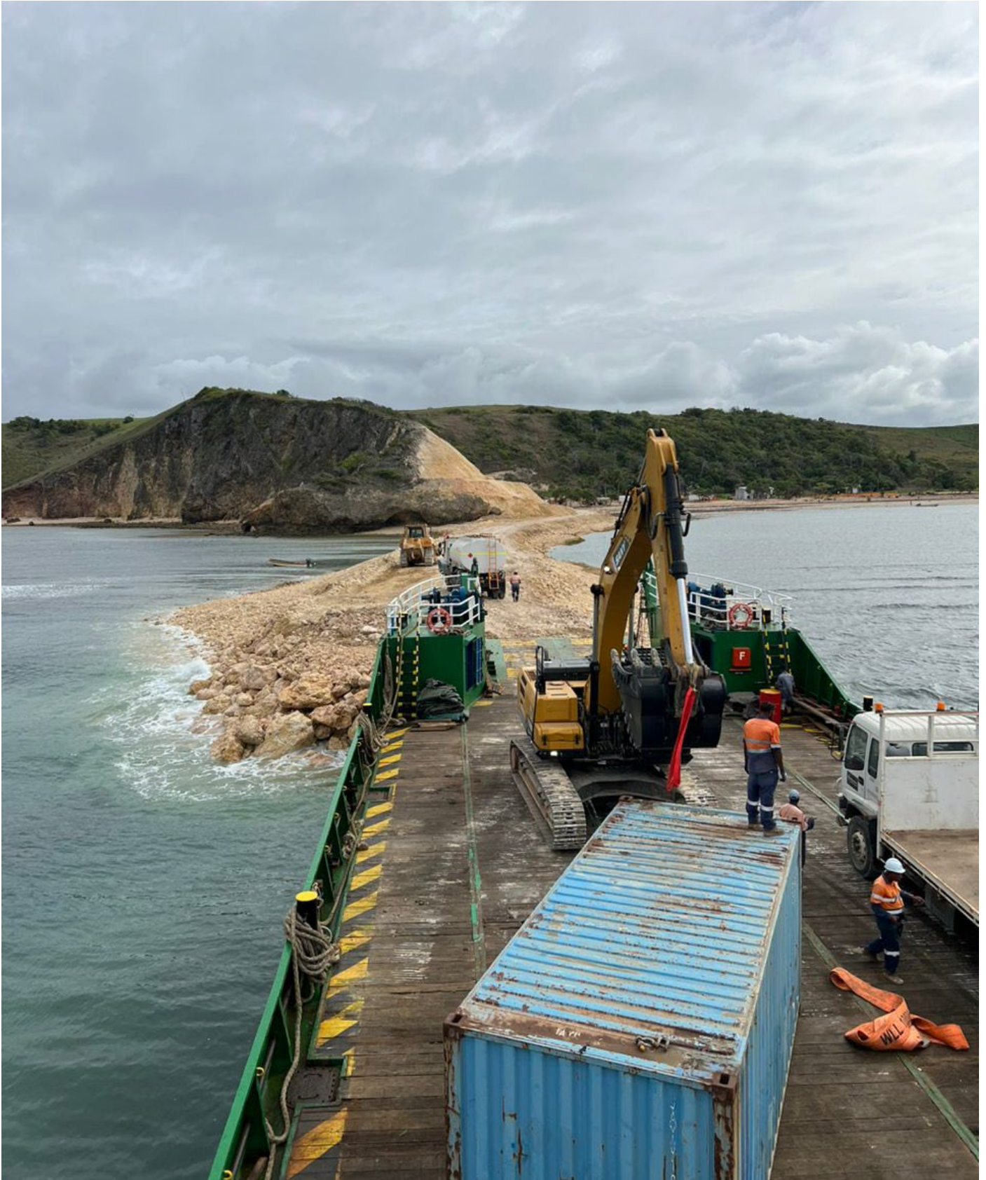
Barge unloading from Wharf
