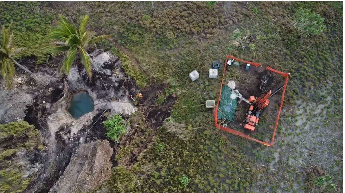
Geotechnical Drill Rig
