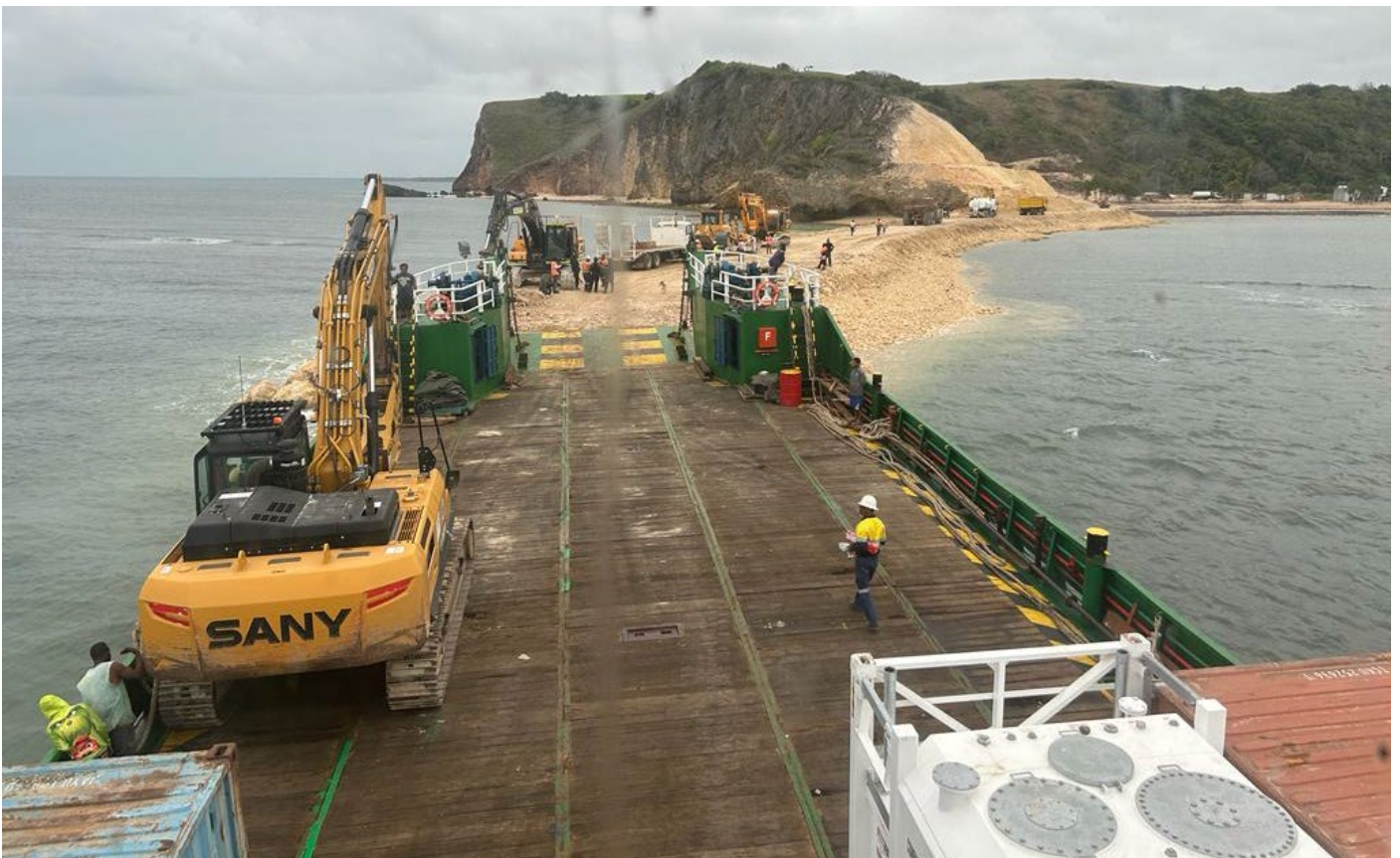
Barge unloading from Wharf
