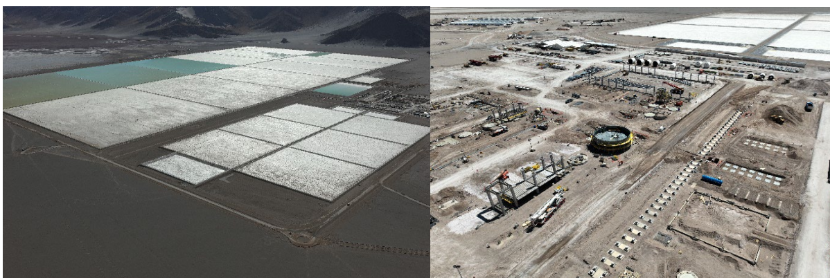
Figure 1: First 2 strings of evaporation ponds complete (left), plant construction underway (right)
