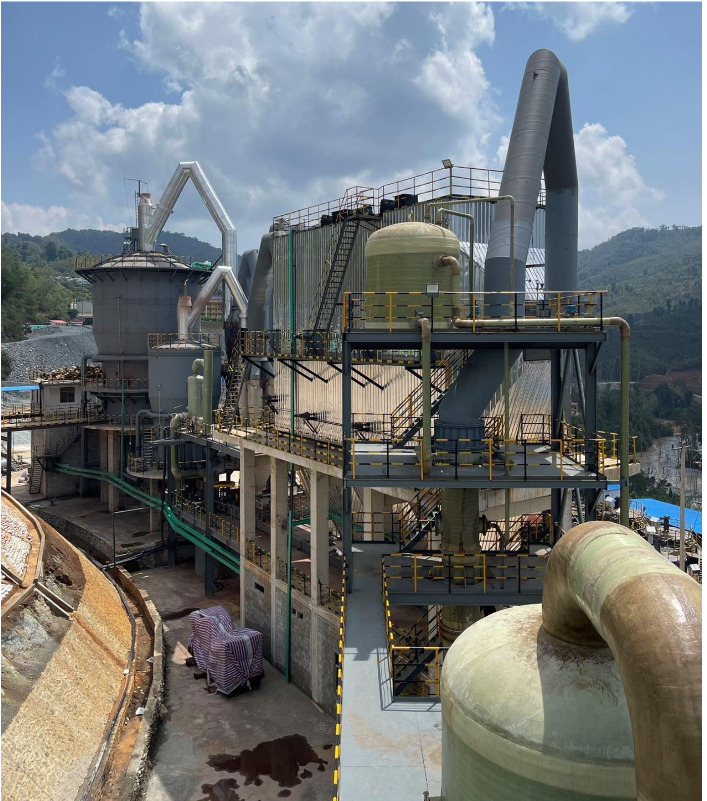
Recently Commissioned 300tpd Two Stage Roaster Ba Mian Gold Mine, Laos
