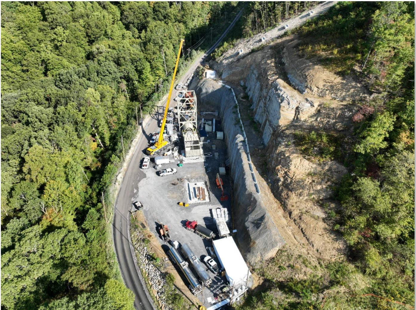
Image: Work commenced on second emission reduction VAM unit – Buchanan Mine
