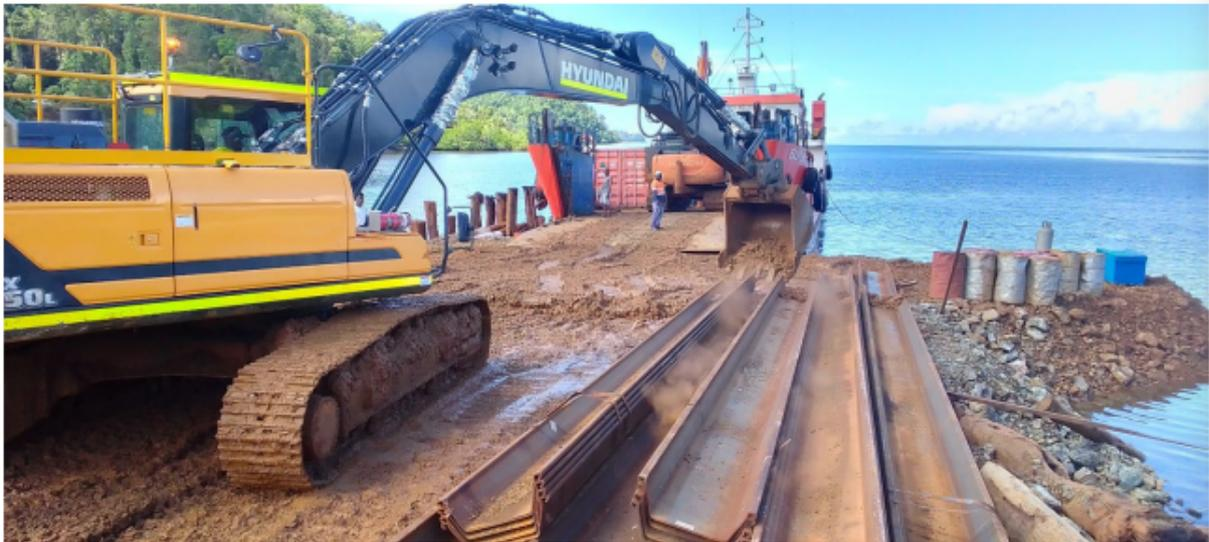
*Sheet piles to be used in construction of the Wharf arriving at Kolosori*
