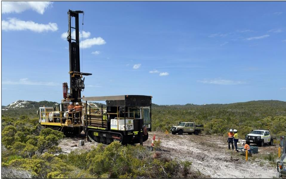
Figure 1: Sonic drilling rig completing groundwater bore drilling
