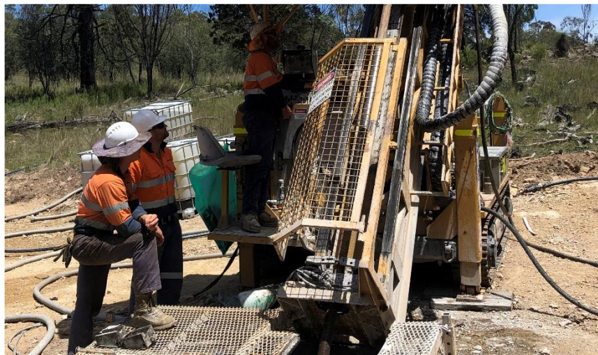
Photo 2 – Drill rig at Webbs Consol Silver-Base Metals Project
