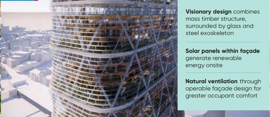
**Visionary design** combines mass timber structure, surrounded by glass and steel exoskeleton
