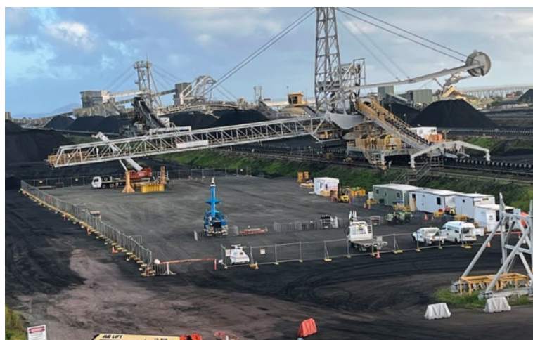
Figure 15: ST1 deconstruction before and after
