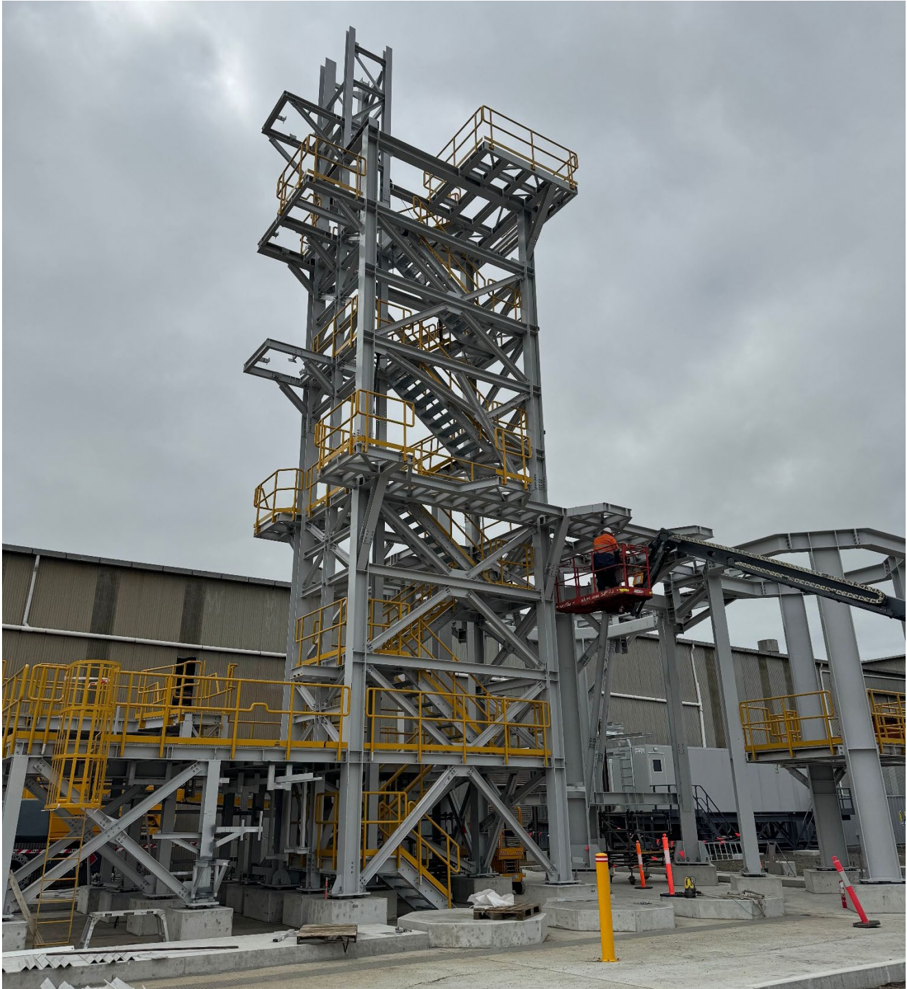
Figure: Spray Raster Structural Steelwork complete to receive Reactor Vessel
