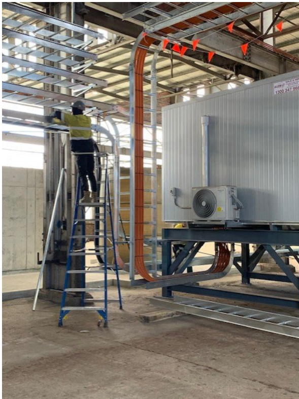
Figure: Electrical and instrumentation cable installation in cable trays & local junction boxes
