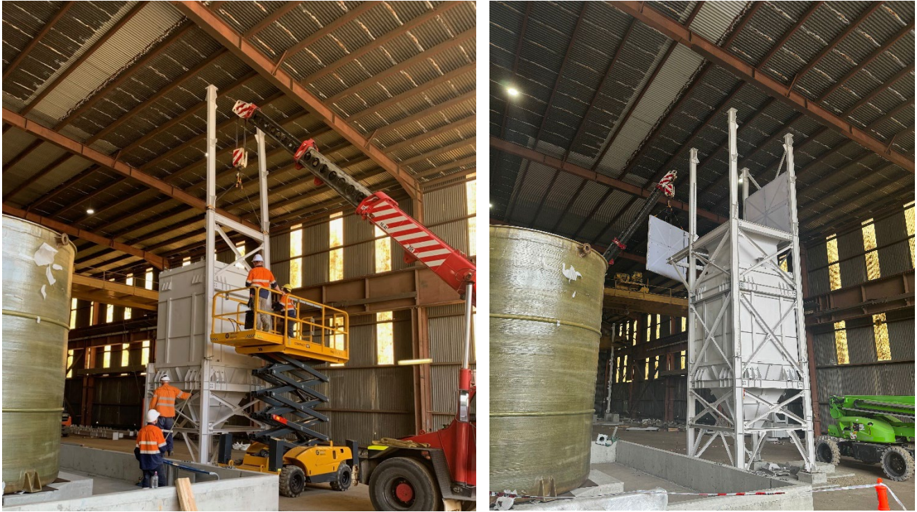
Figure: Magnesite Hopper & Bag Breaker erection
