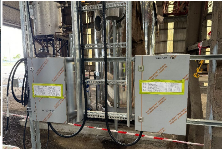
Figure: Electrical and instrumentation cable installation in cable trays & local junction boxes
