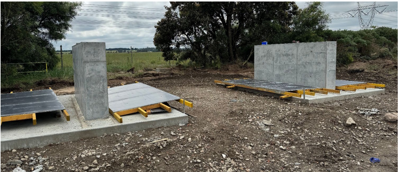
Figure: LPG tank concrete footings completed
