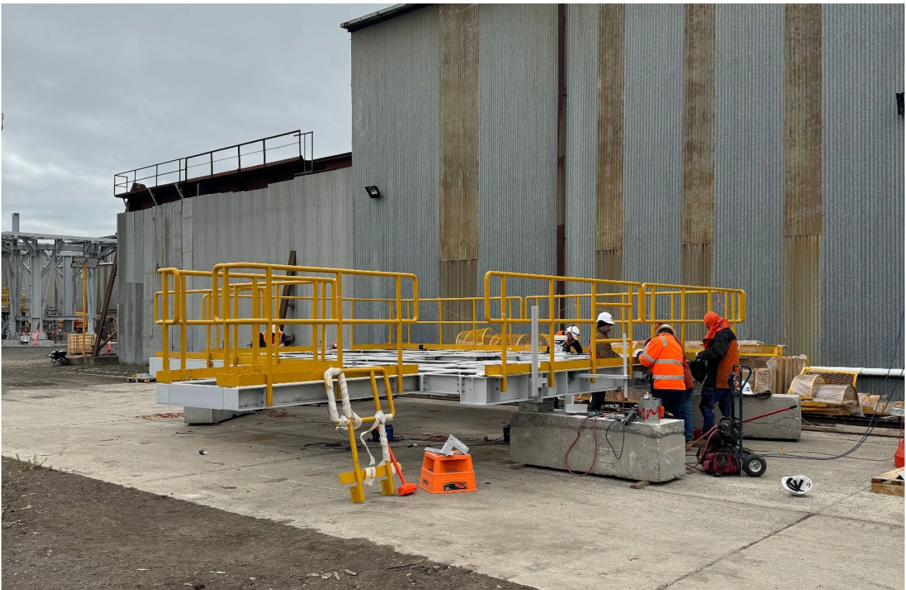
Figure: Assembly and erection of modularised Spray Roaster structural stair tower (top) & platform (bottom)
