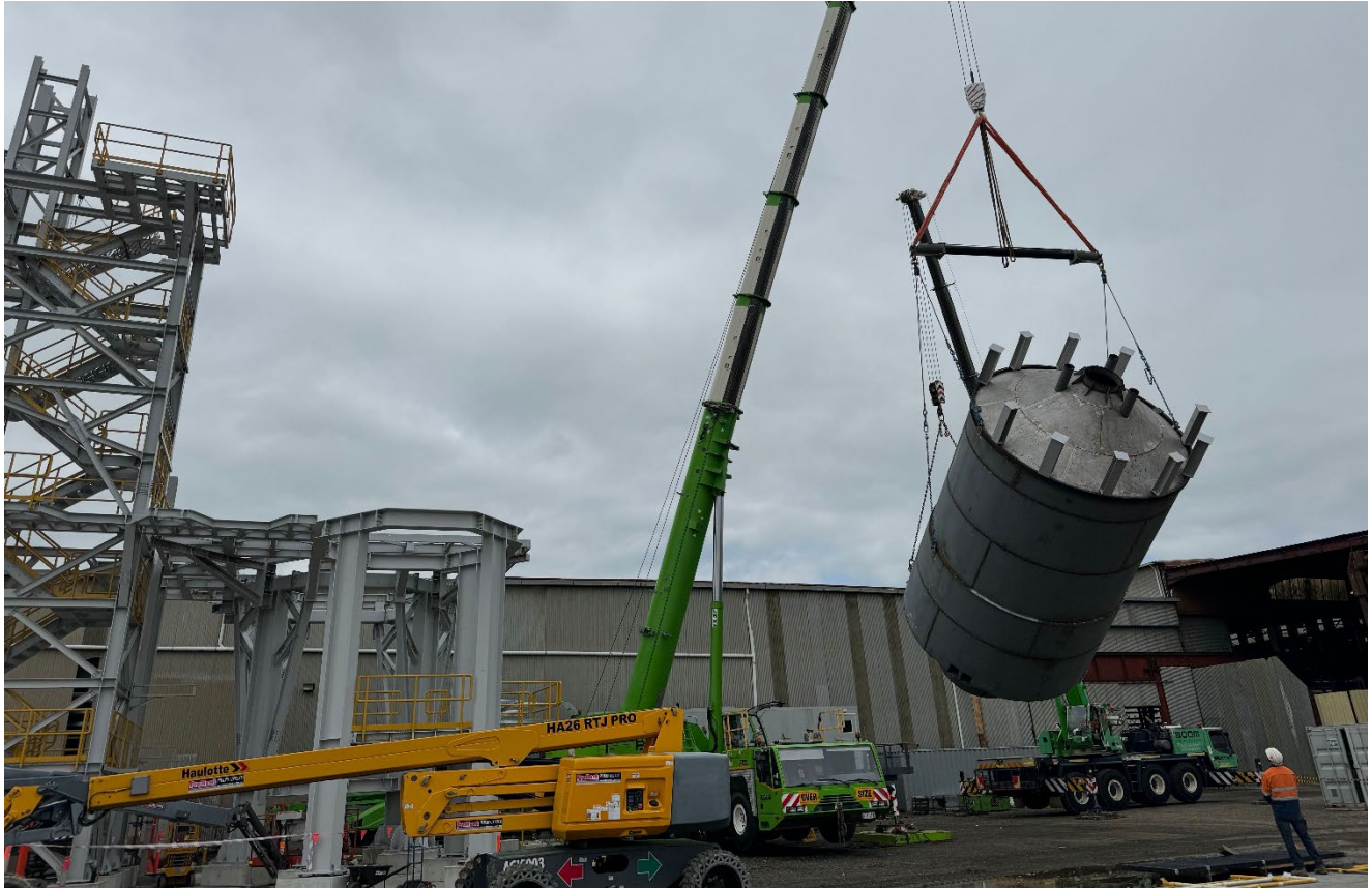
Figure: Spray Roaster reactor vessel dual crane lift
