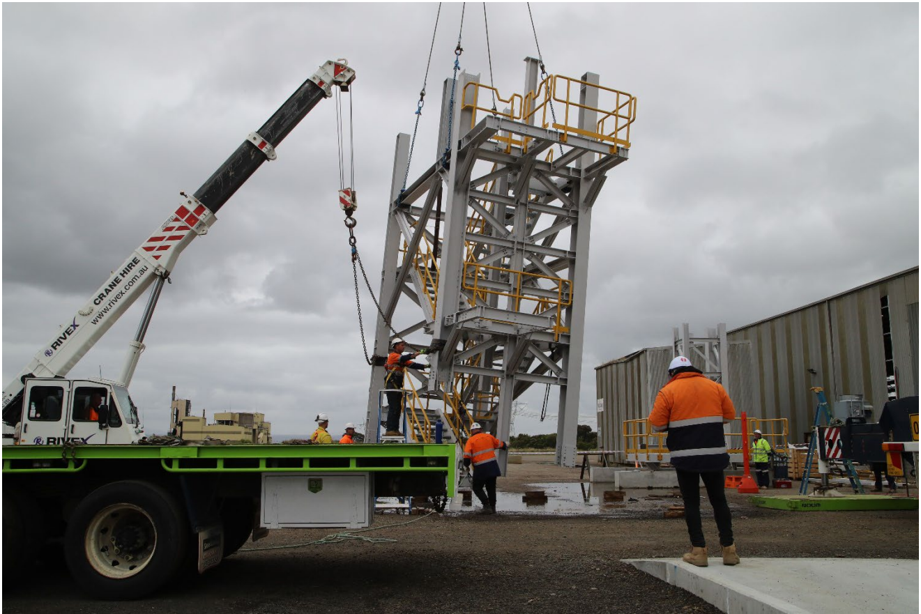
Figure: Assembly and erection of modularised Spray Roaster structural stair tower (top) & platform (bottom)
