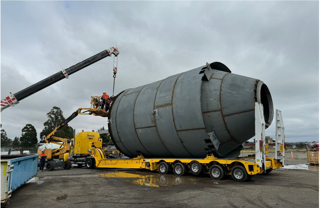
Figure: Spray Roaster reactor vessel transported to site
