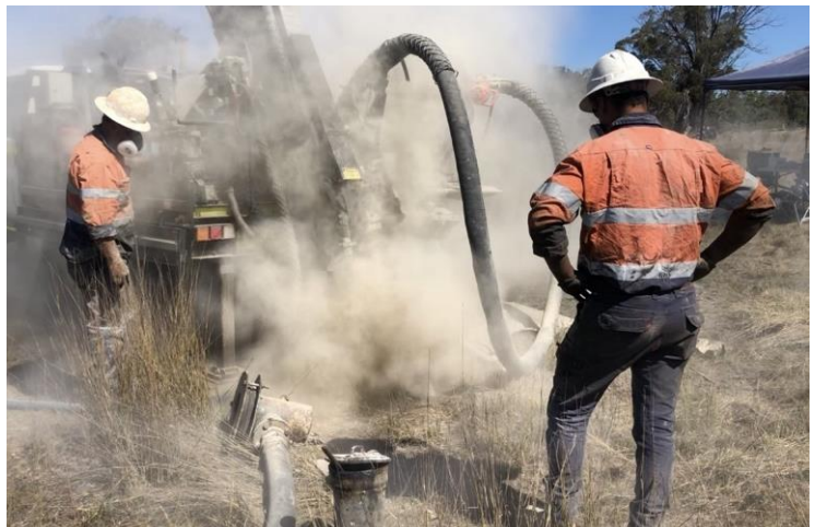
Photo 1. Drilling commences at Webbs Consol North
