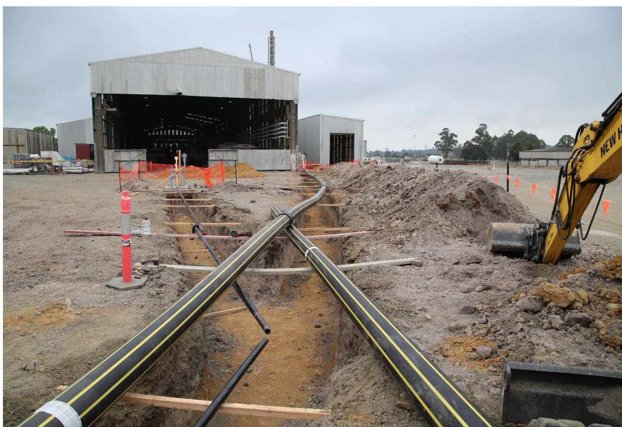
Figure: Origin LPG bullet and underground pipeline being installed
