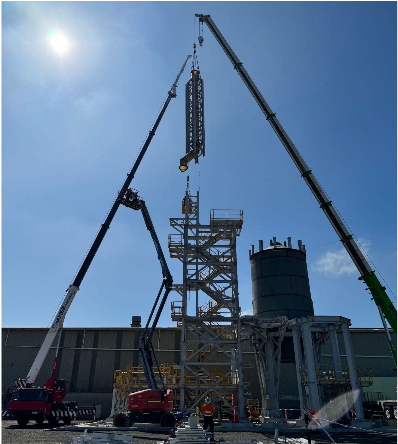
Figure: Installation of modularised Spray Roaster Stack structural steel with piping
