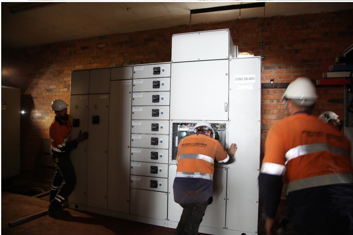
Figure: Electrical and instrumentation cable installation & main switchboard (MSB) replacement
