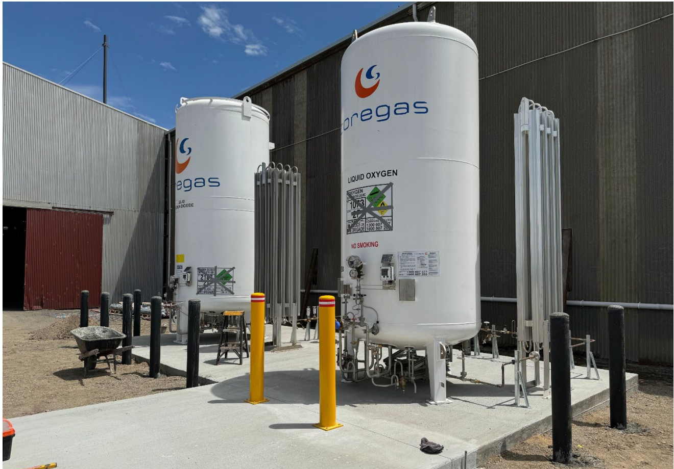
Figure: Coregas oxygen and carbon dioxide system installed
