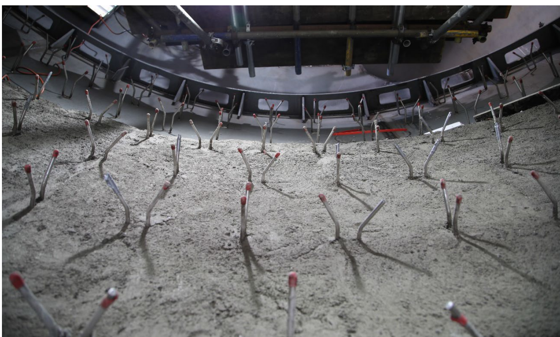
Figure: A close-up of the internal refractory lining of the reactor vessel
