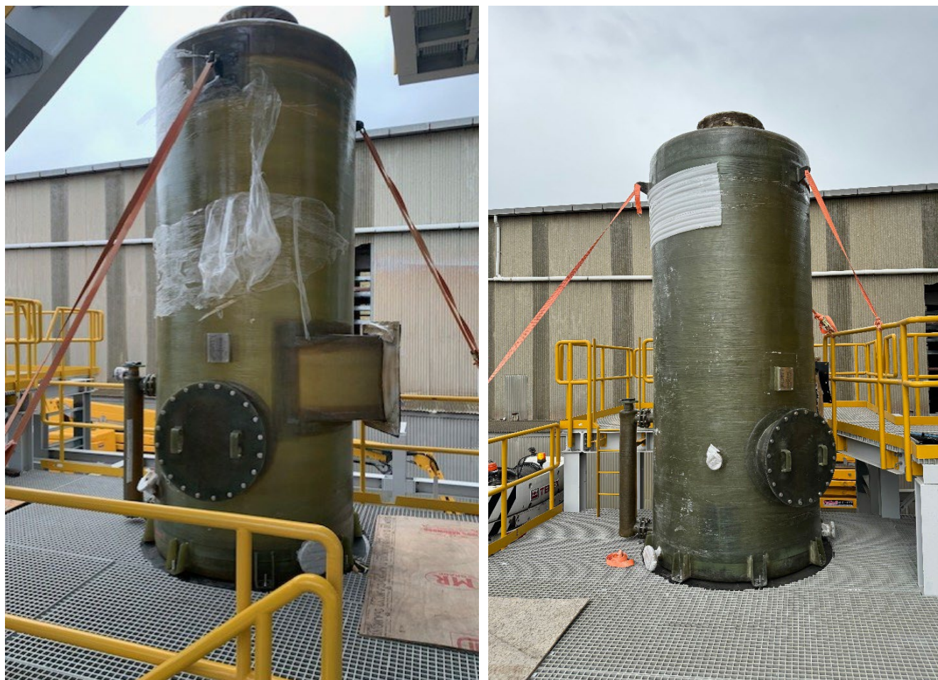
Figure: Spray Roaster tanks installed in final position
