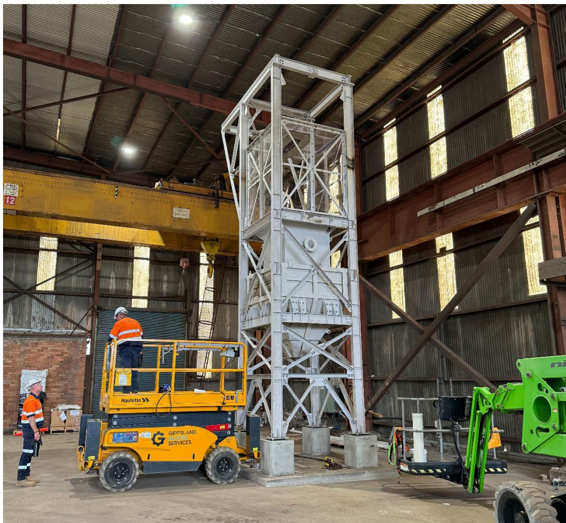
Figure: Ferrosilicon Bag Breaker erection complete
