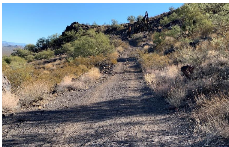
Existing Road leading to Mines
