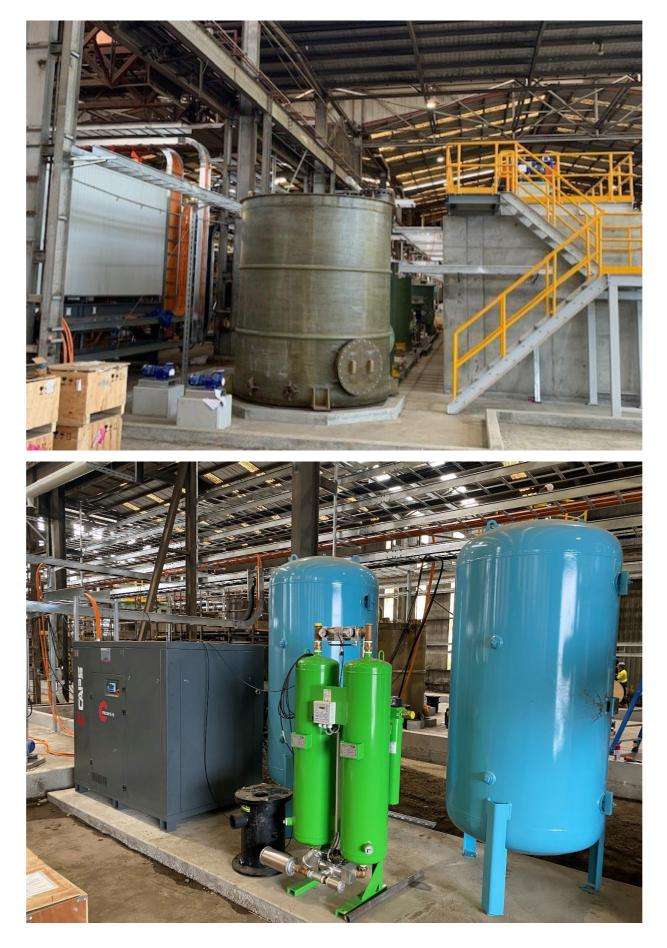
Figure: Filter area FRP tanks and air compressors installed
