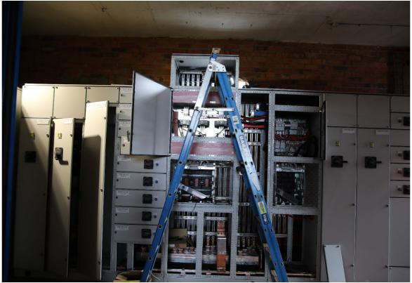
Figure: New Main Switchboard (MSB) installed and powered.
