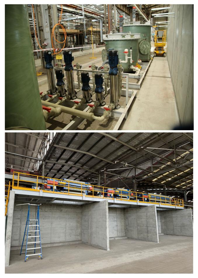
Figure: Filter Presses installed over Filter bunkers and all major mechanical equipment
