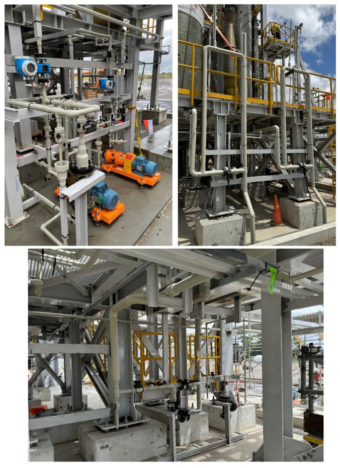
Figure: Piping, valves, and instrumentation installation progressing
