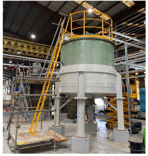
*Figure:* Thickeners with internal rakes installed (top) and carbon steel spools welded ready for install (bottom)
