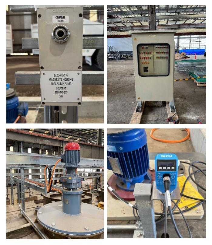
Figure: Installation of local control stations, electrical cabinets and instrumentation and cabling.
