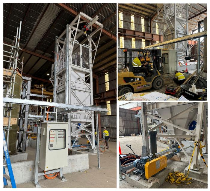
Figure: Magnesite Hopper & Bag Breaker unit E&I and Mechanical equipment installation completed.
