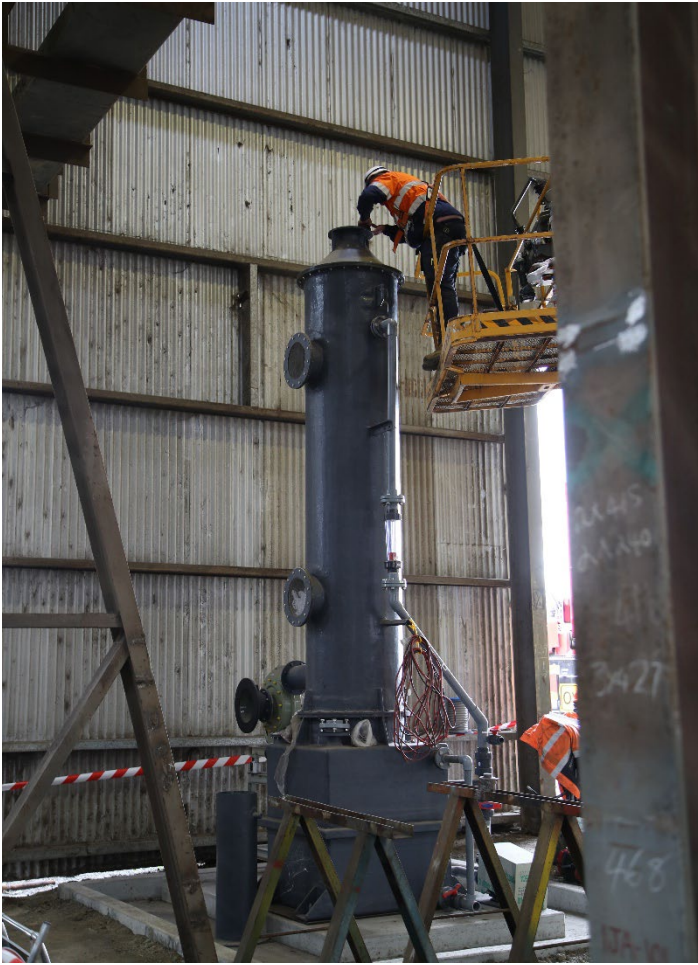
Figure: Erection of Acid Area Scrubber exhaust stack
