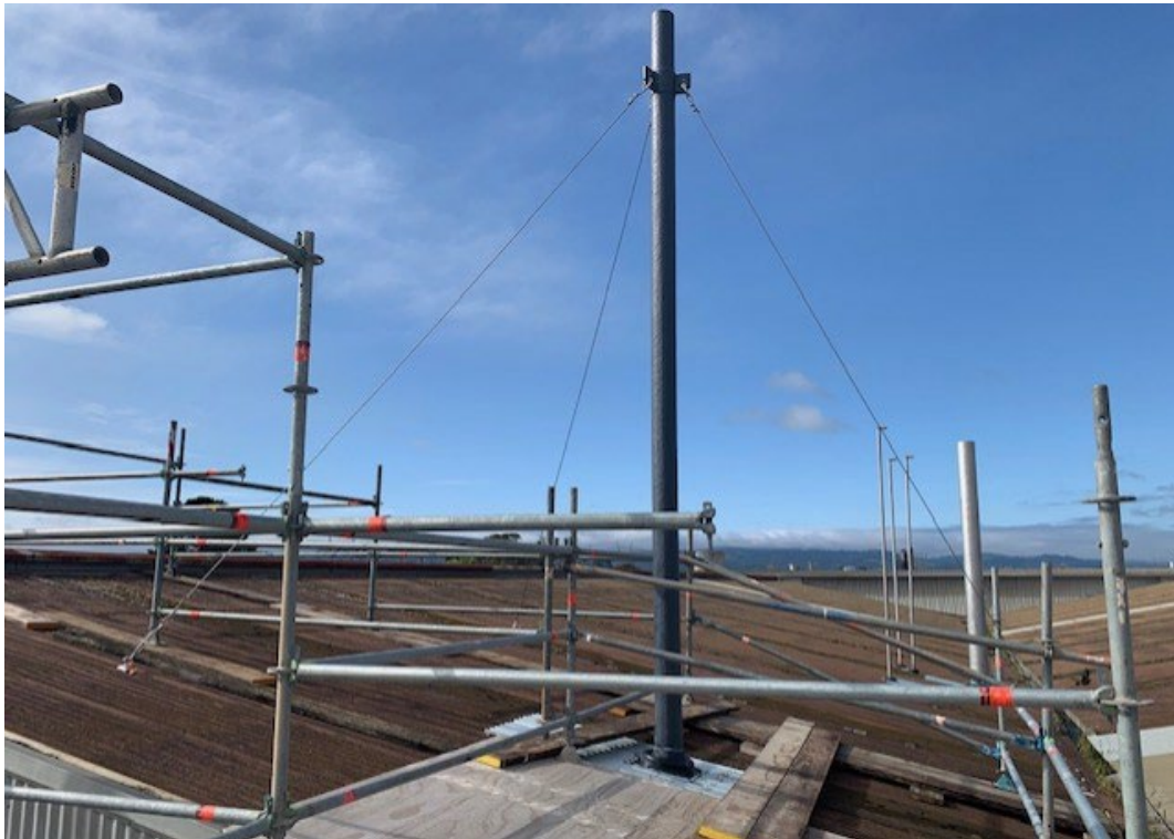
Figure: Erection completion for Acid Area Scrubber exhaust stack
