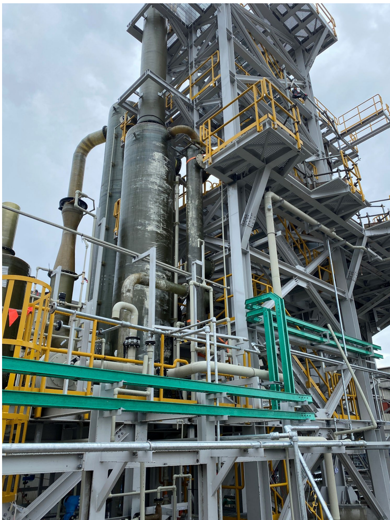
Figure: Mechanical and piping installation progressing
