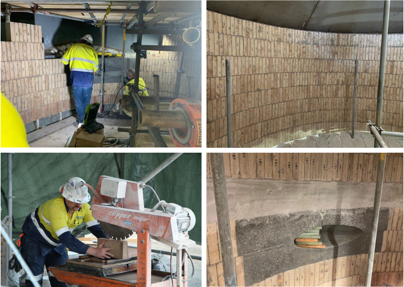
Figure: Spray Roaster reactor vessel refractory lining completed.
