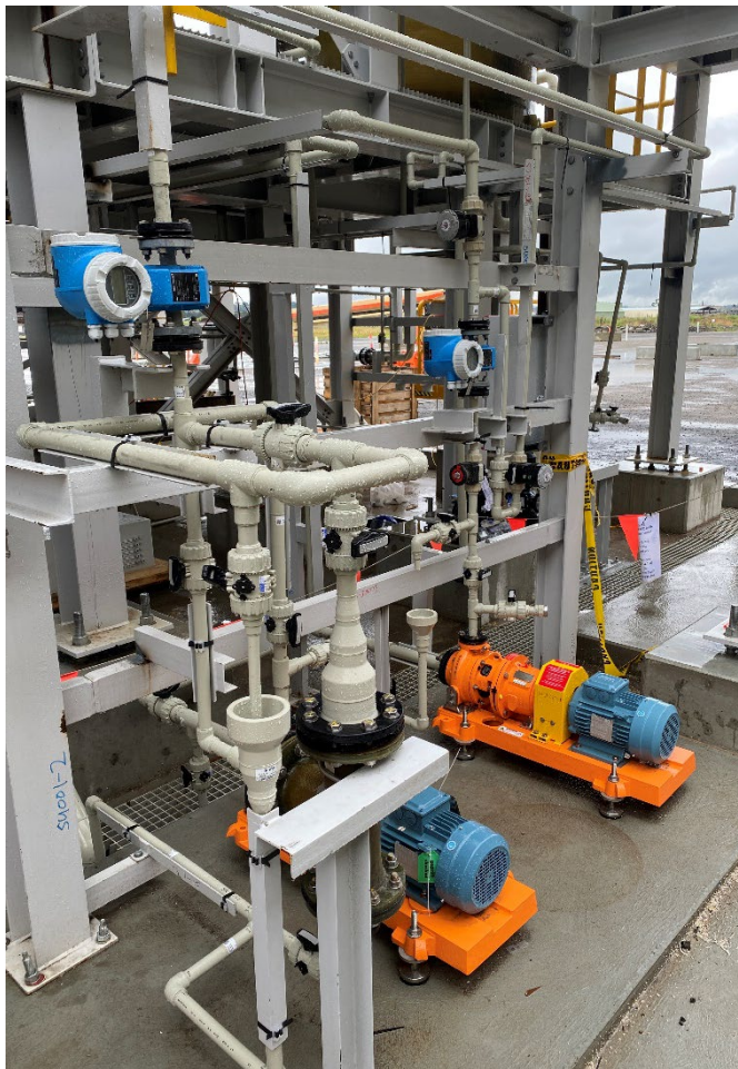
Figure: Spray Roaster tanks, piping, valves, and instrumentation installation progressing
