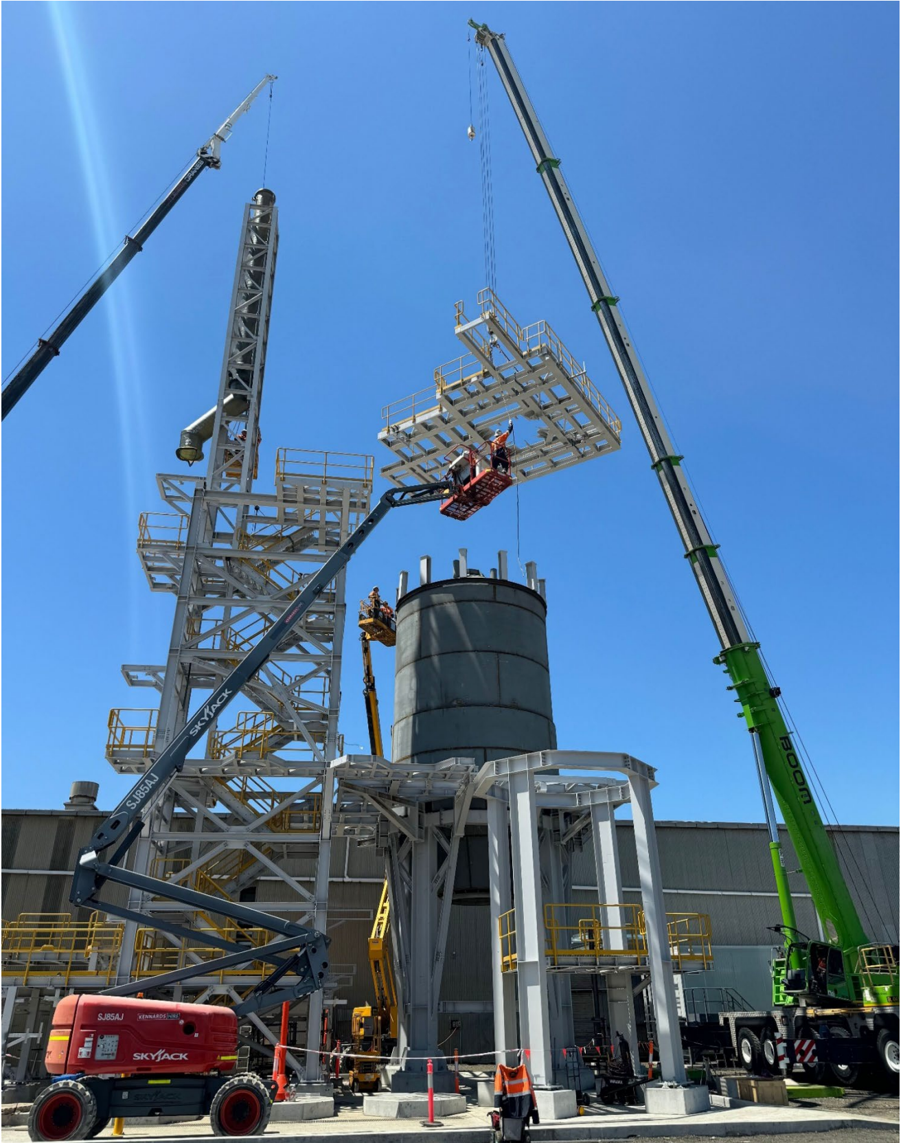
Figure: Installation of modularised Spray Roaster structural steel platforms
