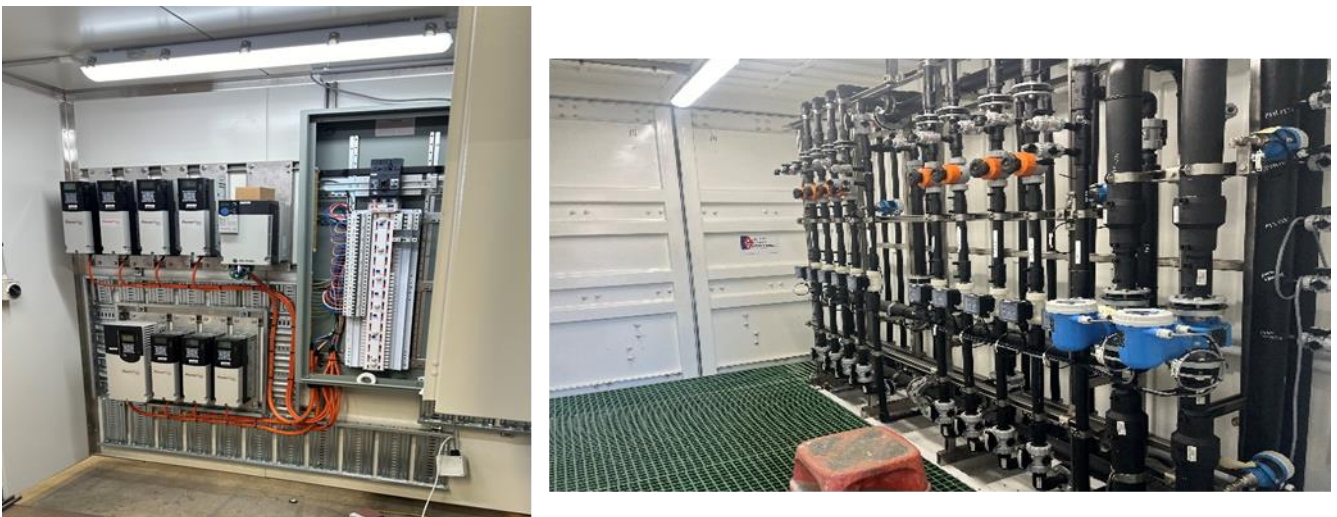
Figure 4: Completed wellhouse module.
