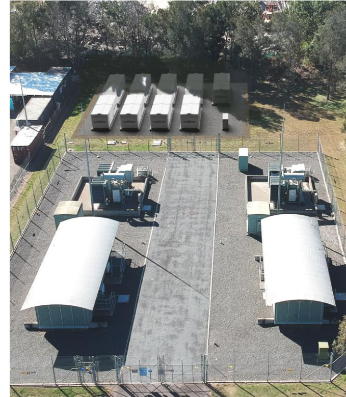
Artist impression of deployment at Energex sub-station at Raceview, Queensland Australia
