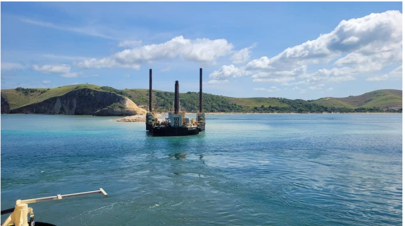
Jack up rig Jake 1 in position and commencing jack up, December 2023
