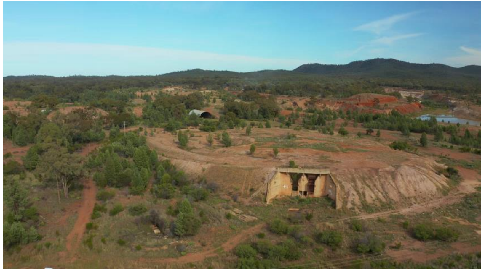
Drone over the Tallebung Tin Mining Field – Old Crusher and ROM to Southern Open Pit
