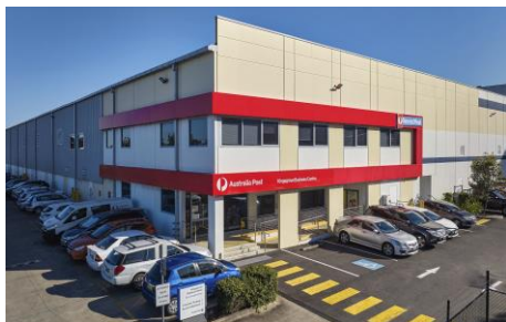
Australia Post, Kingsgrove NSW
