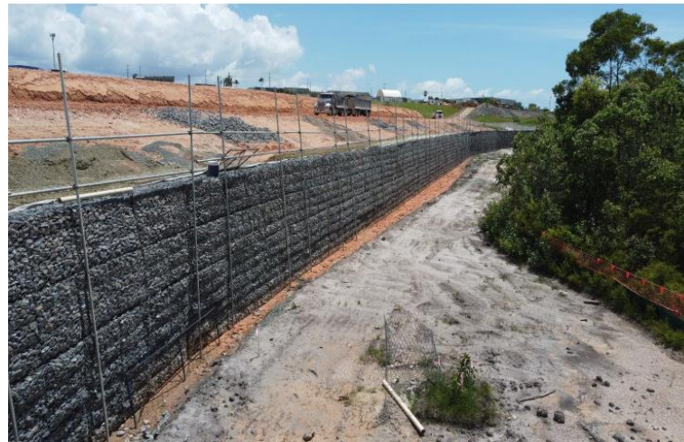
B 800 metre retaining wall construction progress
