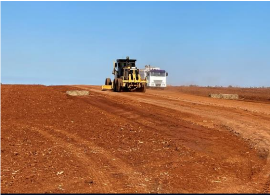
Initial ground preparation at Dowlings, Maryborough, Queensland, October 2021.
