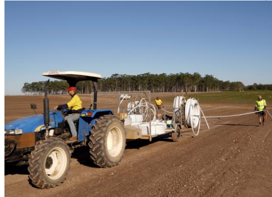
Laying infield irrigation pipe at Dowlings, Maryborough, Queensland, May 2023.
