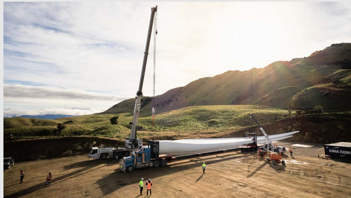
Blade transportation at Meridian's Harapaki wind farm
