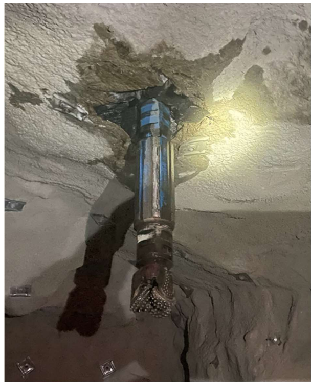
Figure 2: Pilot hole breakthrough
