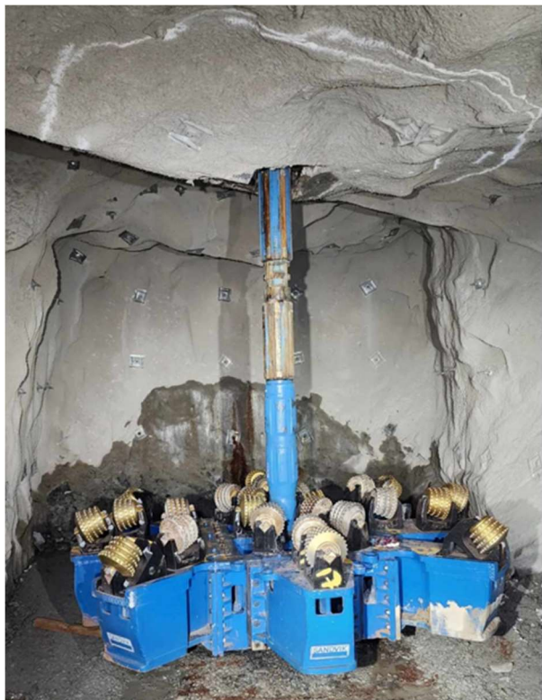
Figure 3: Reamer head being attached to rods
