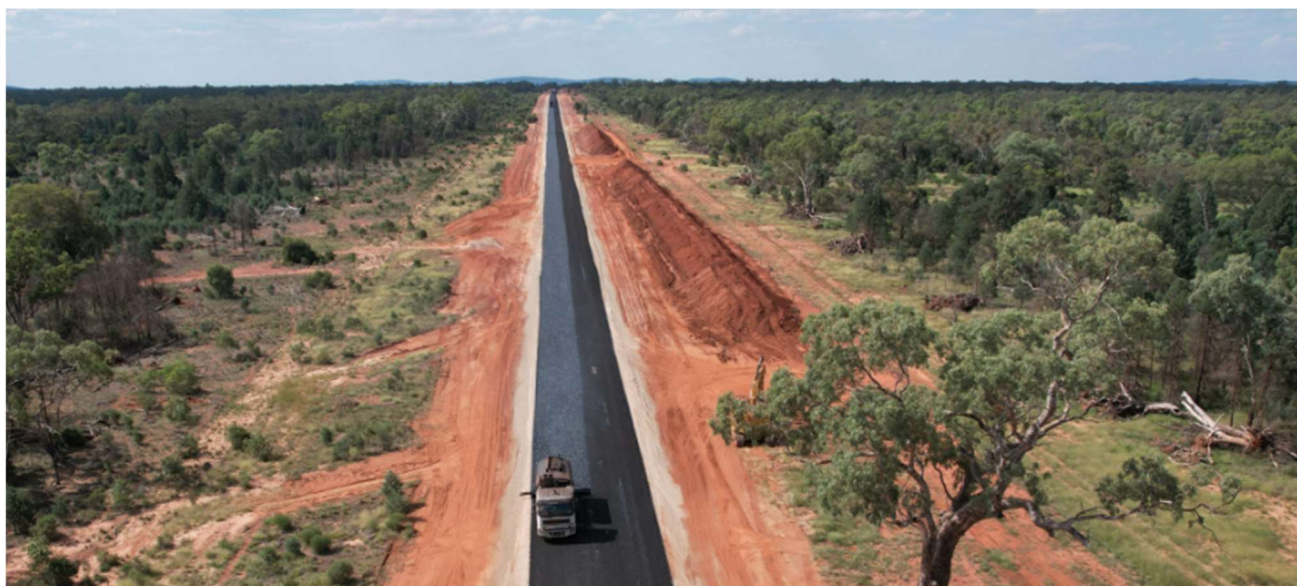
Figure 4: Road sealing works along the Burthong Road.
