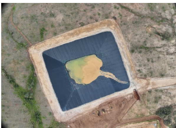
Figure 2: Brine dam commencing operation.
