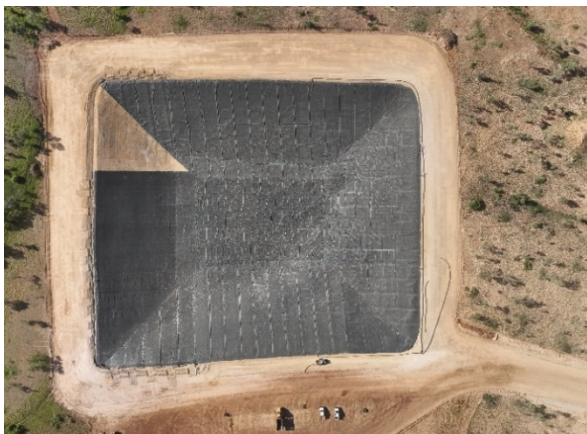
Figure 1: Brine dam nearing completion.
