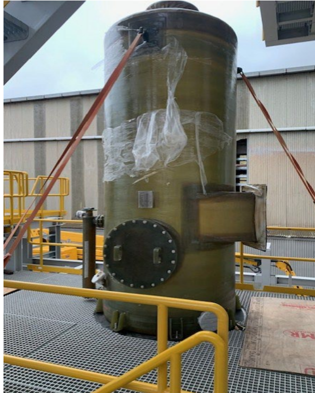
Spray Roaster tanks installed in final position
