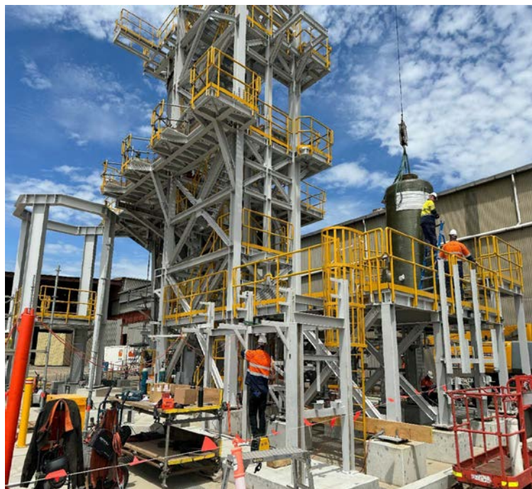
Spray Roaster mechanical equipment installation progressing
