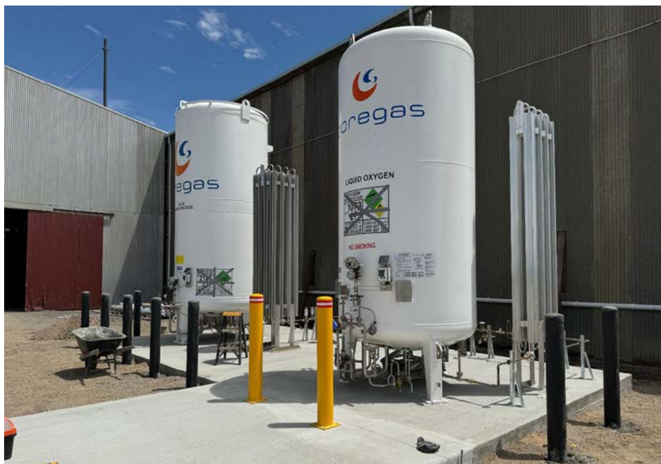
Coregas oxygen and carbon dioxide system installed
