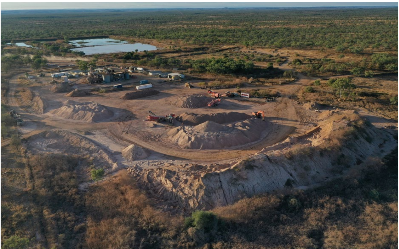
Georgetown Processing Plant and ROM stockpiles
