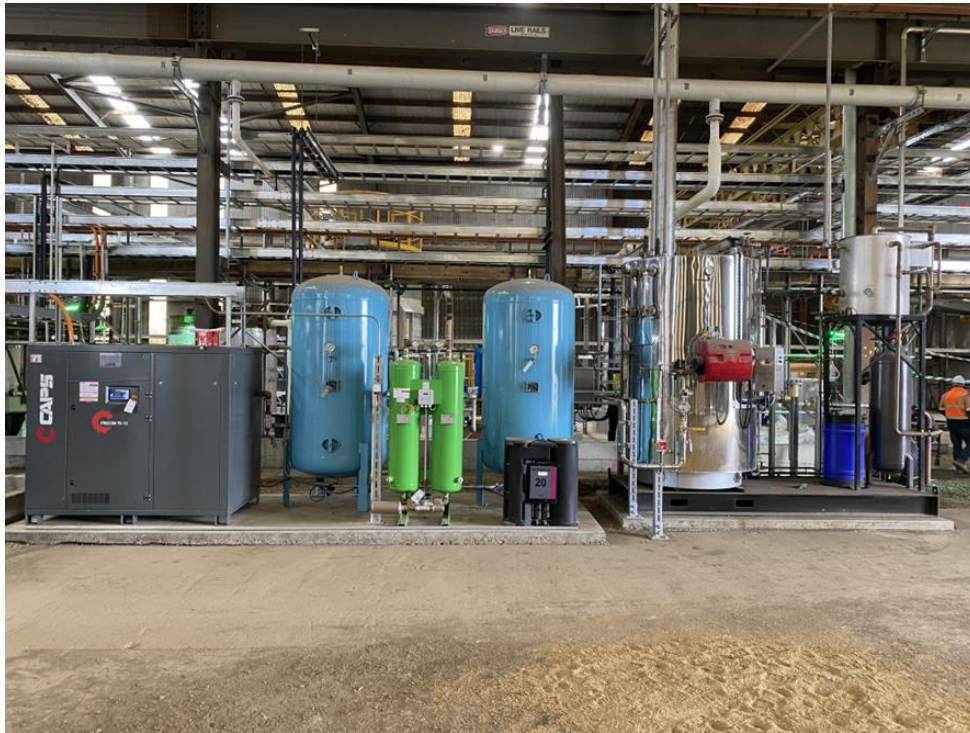
Figure: Process Air, Instrument Air undergoing commissioning
