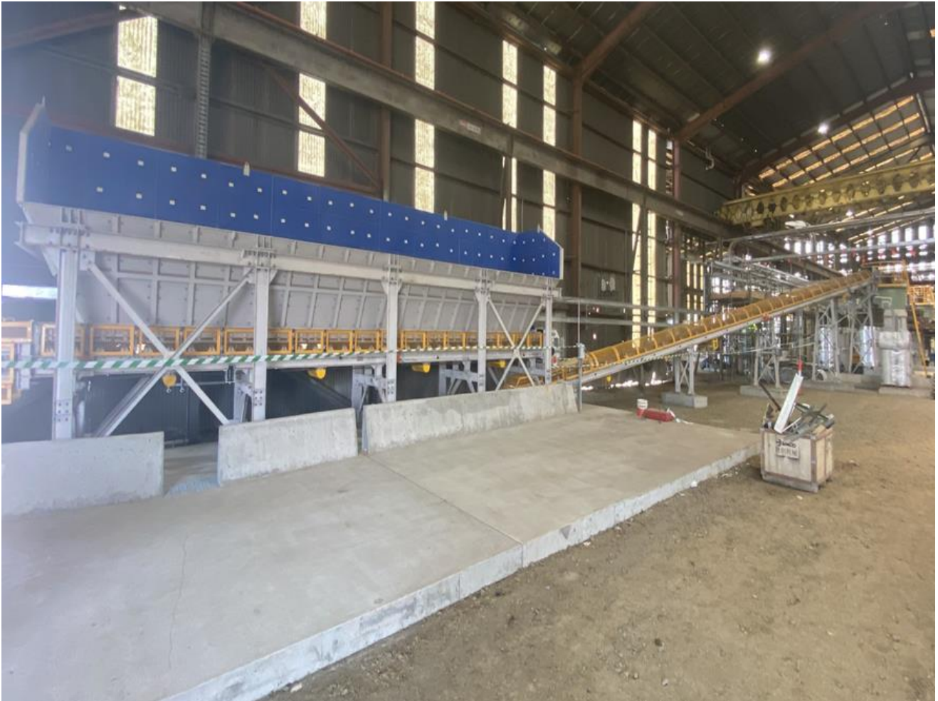
Figure: Ash Handling area complete
