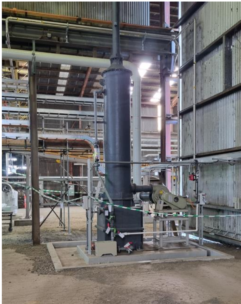
Figure: Acid Scrubber area under commissioning
