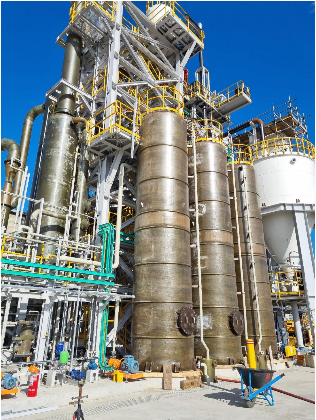
Figure: Spray Roaster mechanical and piping complete
