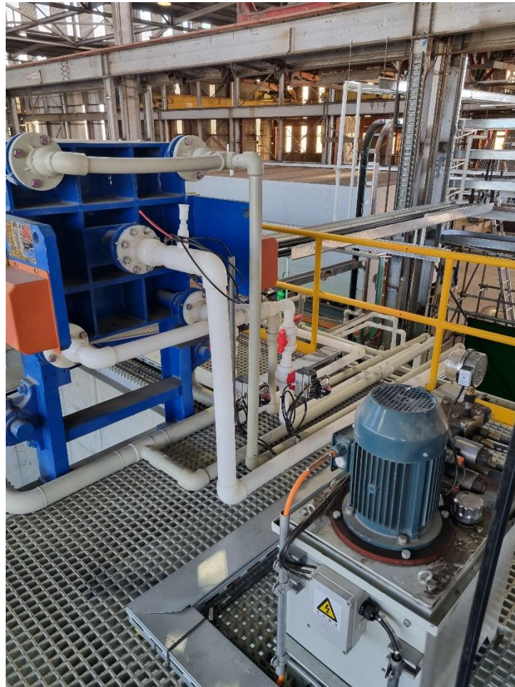
Figure: Filtration piping, hydraulics and electrics installed
