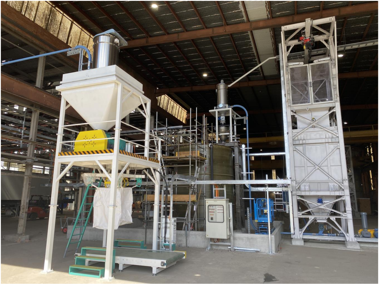
Figure: MgO Bagging Plant completed
