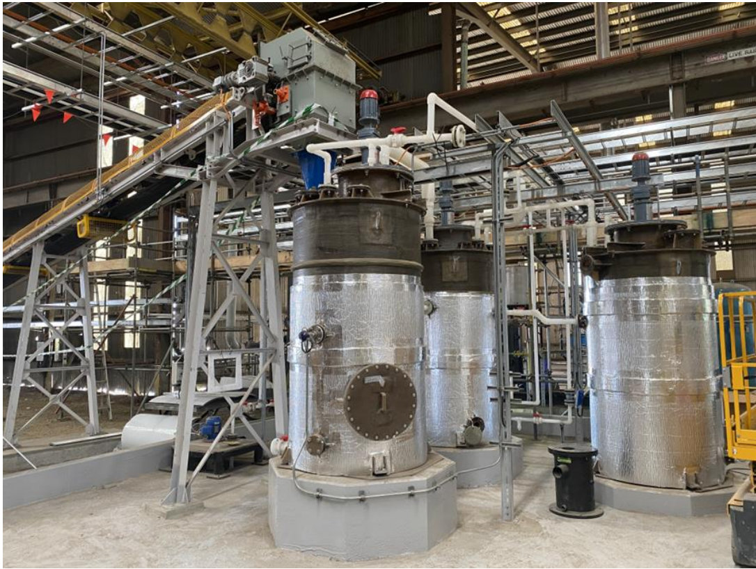
Figure: Acid Leach area complete
