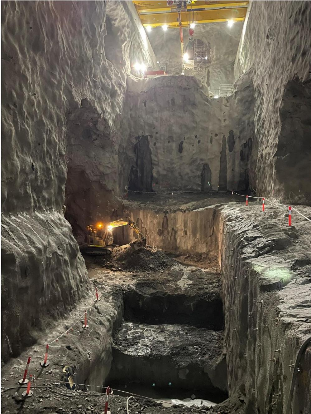
Figure 3: Powerhouse Excavation complete – Looking from CA03 – Opening for Tailrace Tunnel for Unit 2 indicated
