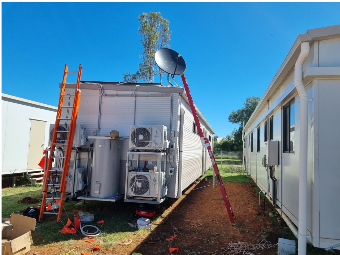
Image 2: Camp Expansion Phase 1 Installation
