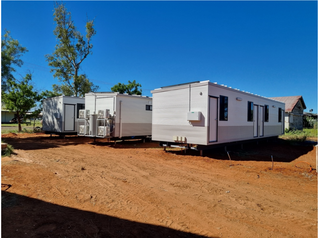
Image 1: Camp Expansion Phase 1 Installation
