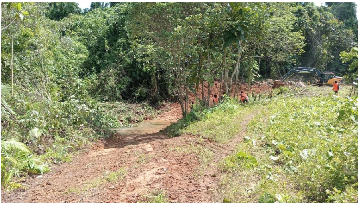
Figure 7 Track construction, Willie Creek, April 2024
