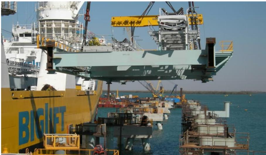
*Figure 6: Modular wharf construction using HLS*
