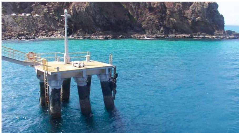
*Figure 29: Mooring dolphin structure consisting of 6 raked piles*
