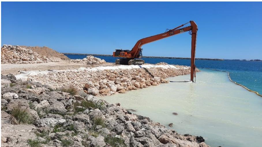
Figure 17: Installation of primary and secondary rock armour on top of geofabric
