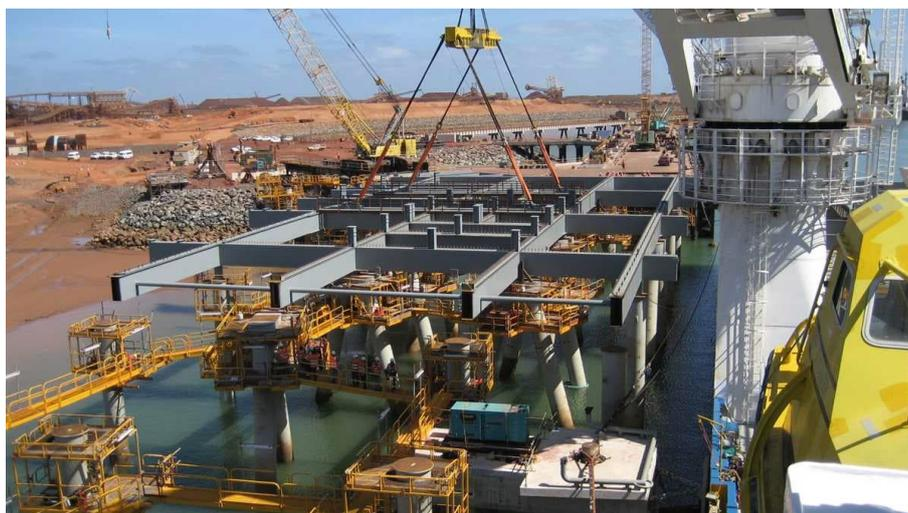
*Figure 31: HLS installing prefabricated deck modules*
