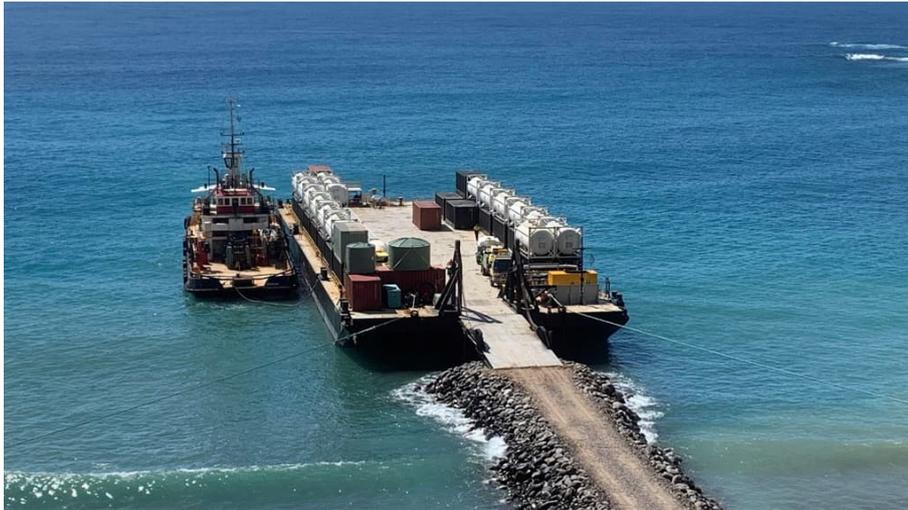
*Figure 5: Temporary barge offloading facility*
