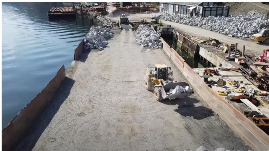
*Figure 13: Typical rock barge being loaded by front-end loader*
