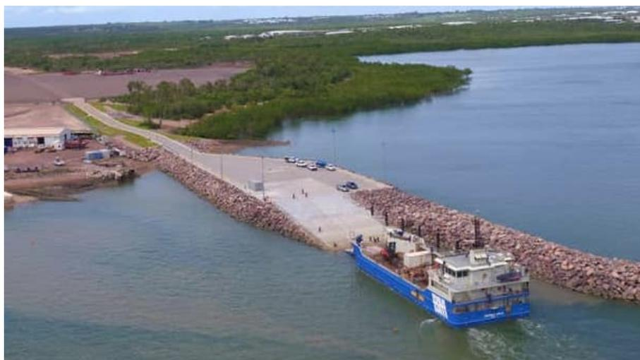
Figure 22: Landing ramp for RORO vessel or landing craft
