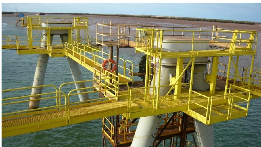
Figure 28: Pile bracing and walkways installed
