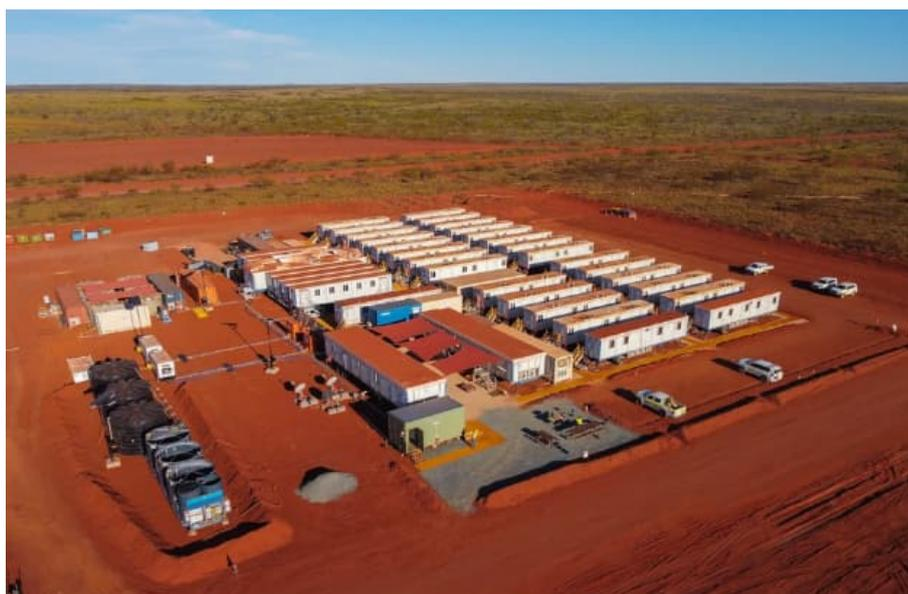
Figure 24: Typical construction camp using transportable buildings
