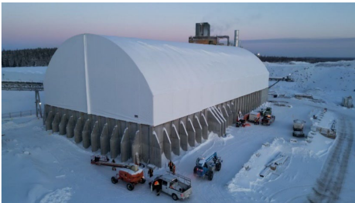
Figures 4 and 5: Crushed Ore Dome final stages of construction
