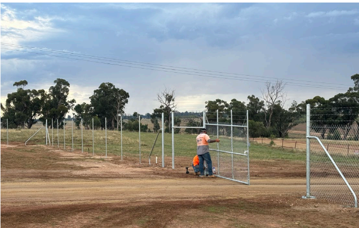
Image 2: Site establishment at Narromine, NSW
