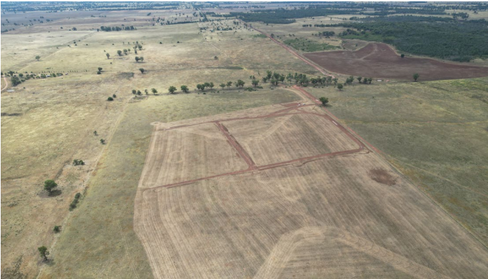
Image 1: Site clearing and access works underway at Narromine, NSW
