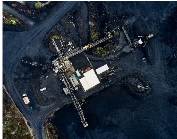
Blair Athol Coal Handling and Preparation Plant
