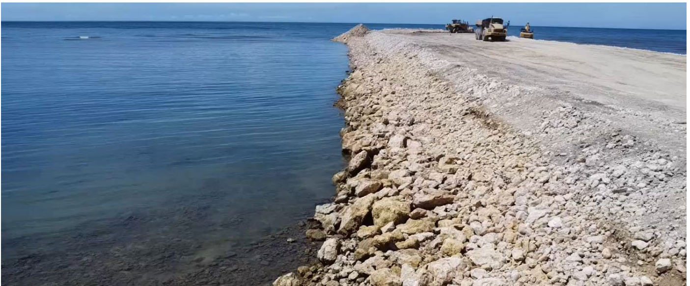
Pioneering Wharf at Central Lime Project
