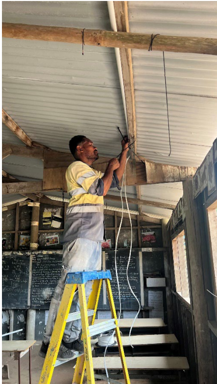
Electrician Completing Installation
